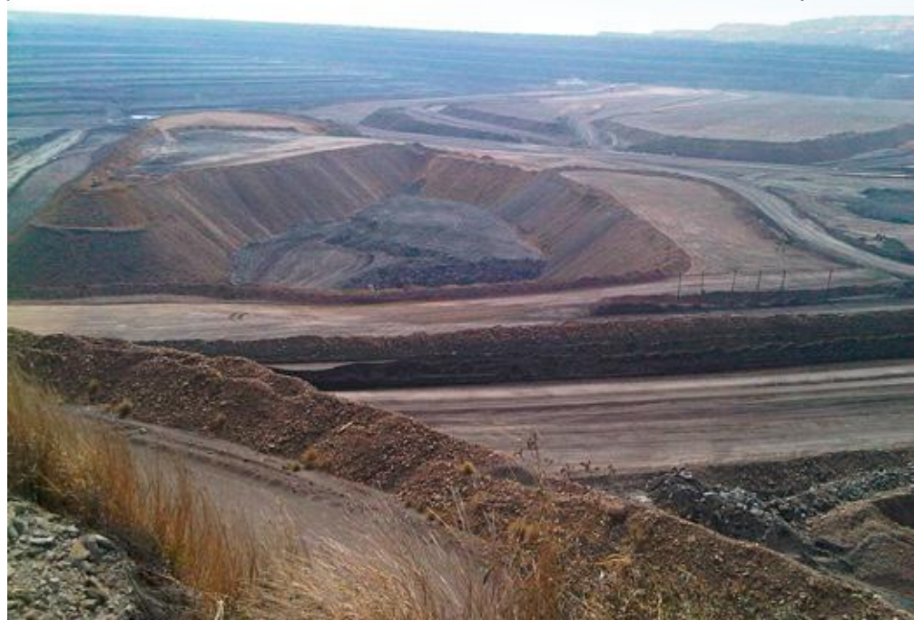
Prepping the site for a Trial Reservoir Project in the UK
