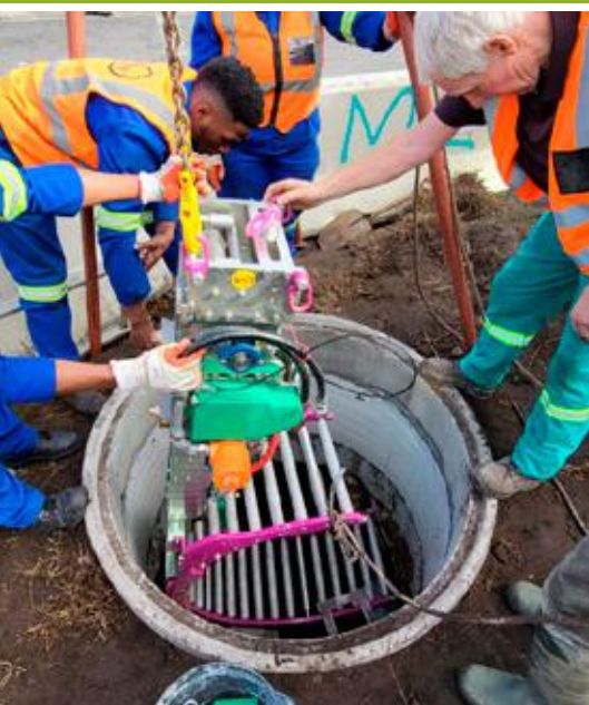
The SWP winding cage and equipment being lowered into a manhole
