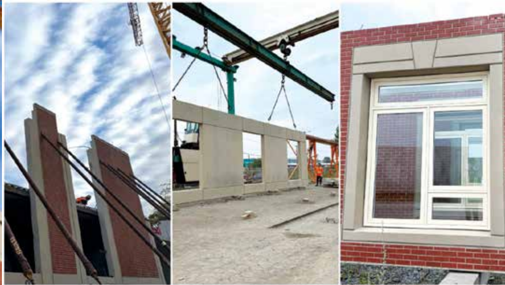
Left: Instead of traditional cast-in-place concrete, Strescon fabricates and cures individual concrete elements – structural components and exterior enclosures alike – in a factory and then ships them to the site on flatbed trucks for installation. Above: Because the windows arrive pre-installed in the panels, the building is effectively enclosed as the structure rises, avoiding the drafts and temporary hoarding common in winter construction and allowing other trades to move in once the precast is two floors ahead.
