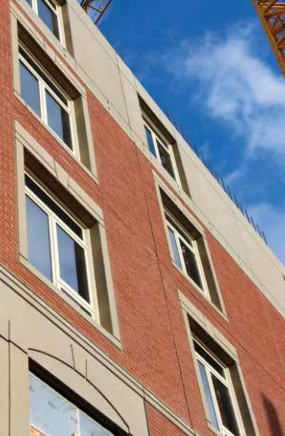
Left: Instead of traditional cast-in-place concrete, Strescon fabricates and cures individual concrete elements – structural components and exterior enclosures alike – in a factory and then ships them to the site on flatbed trucks for installation. Above: Because the windows arrive pre-installed in the panels, the building is effectively enclosed as the structure rises, avoiding the drafts and temporary hoarding common in winter construction and allowing other trades to move in once the precast is two floors ahead.
