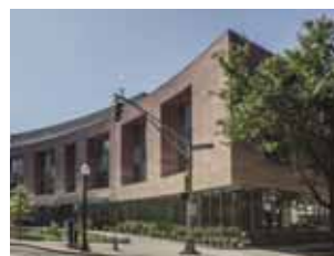
King Open School, Cambridge, MA. Architects: William Rawn Associates, Boston, MA
