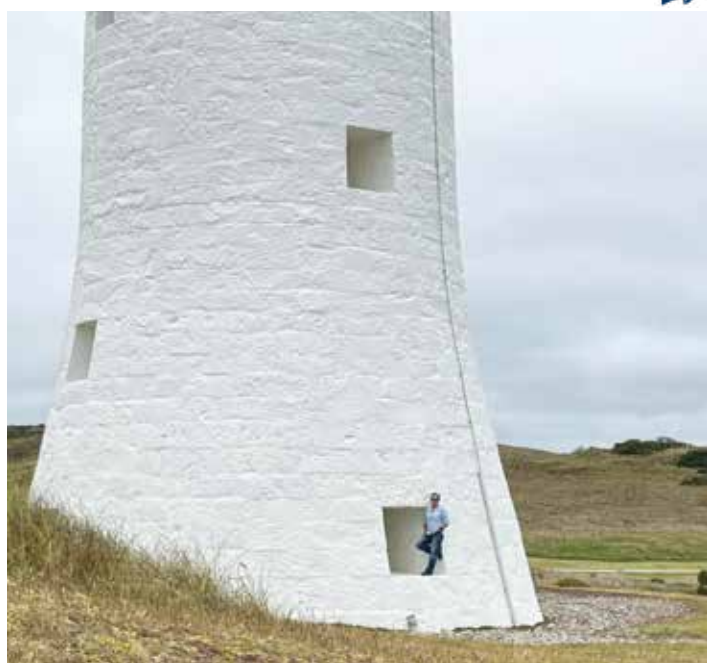
Cape Wickham Lighthouse, King Island. Massive 3.4m thick walls and a height of 48m, Australia's tallest lighthouse.
