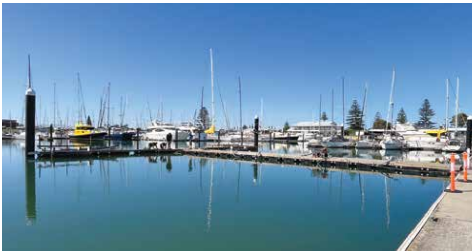
Newly installed BC Row walkway
