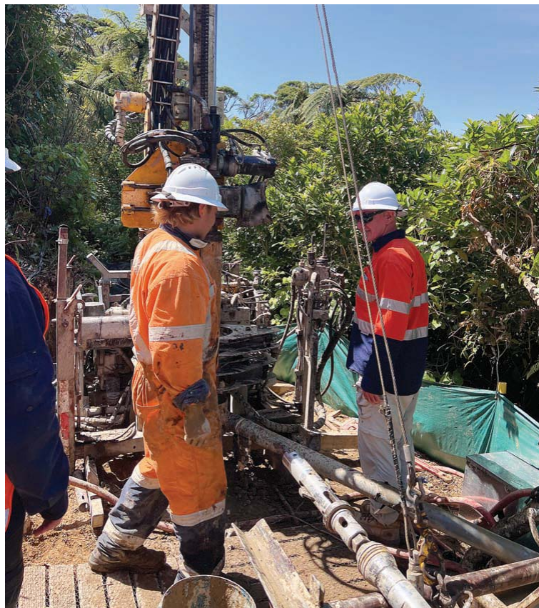
MS workers on a rig on site. Photo: NZTA.
