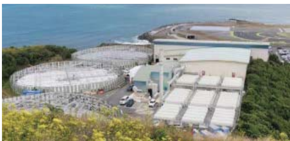
Mōa Point sewage plant. Photo Supplied.
