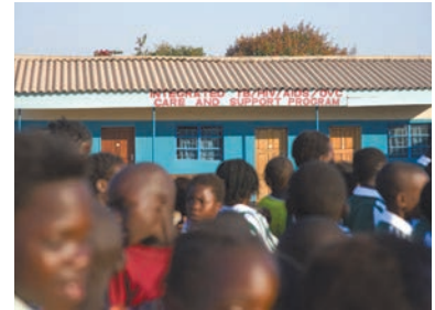
D A new AIDS hospital in Lusaka, Zambia
