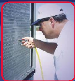
Blow off coils with Sludge Sucker® Blowgun
