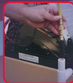
Clean out condensate drain lines with Sludge Blaster®
