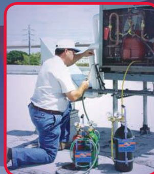
Purge and pressure test an A/C&R system
