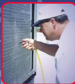
Blow off coils with Sludge Sucker® Blowgun
