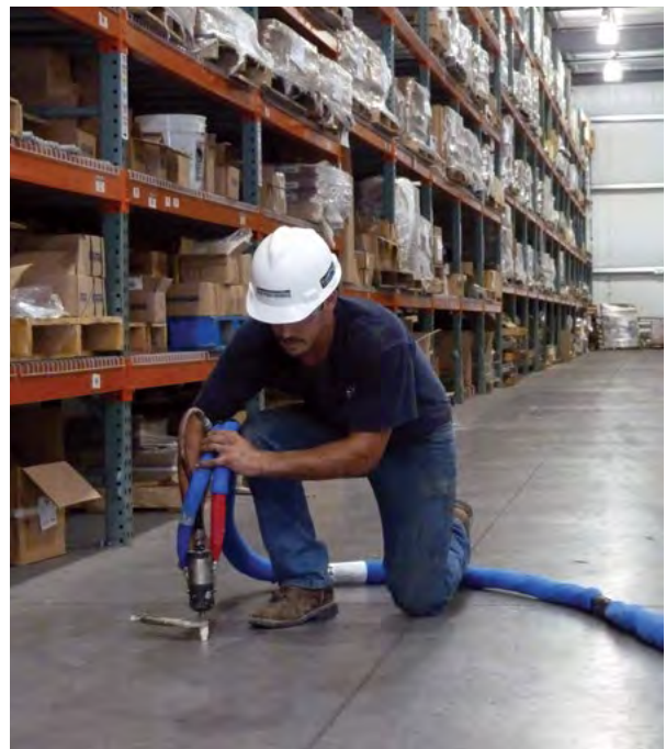
Figure 5.6 PolyLevel stabilizes warehouse floor slab
