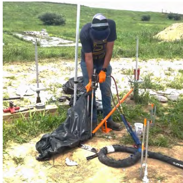
Figure 5.20 Injecting PolyLevel Soil Improvement foam into soil
