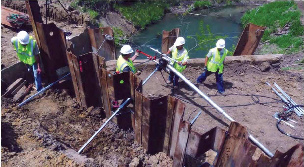
Figure 1.5 Helical tieback installation with hand-held equipment
