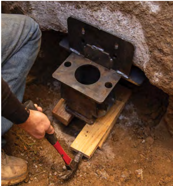
Figure 2.23 Temporary bracket support with wood cribbing
