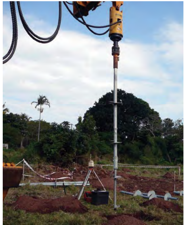
Figure 1.35 Combination pile with HA175 stinger coupled immediately to 3.5" O.D. shaft
