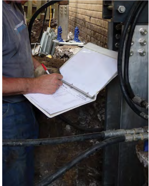
Figure 2.36 Pressure readings are recorded for each pier tube
