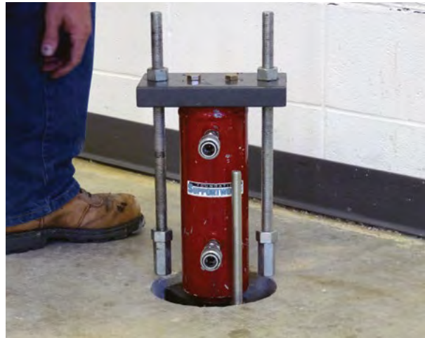
Figure 2.76 Lift cylinder assembly set on pier cap
