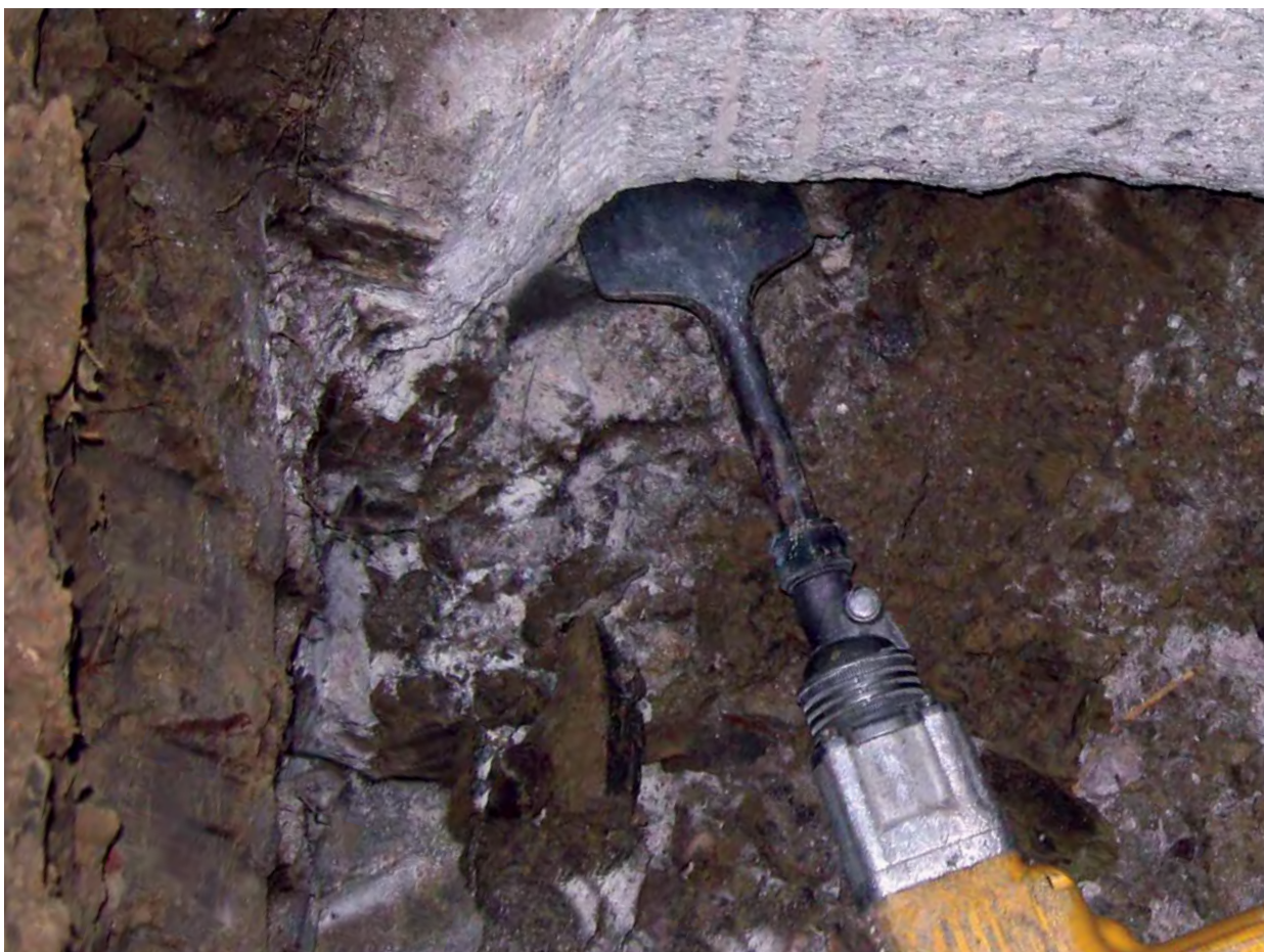
Figure 2.19 Removing soil from beneath the footing with a chisel attachment
