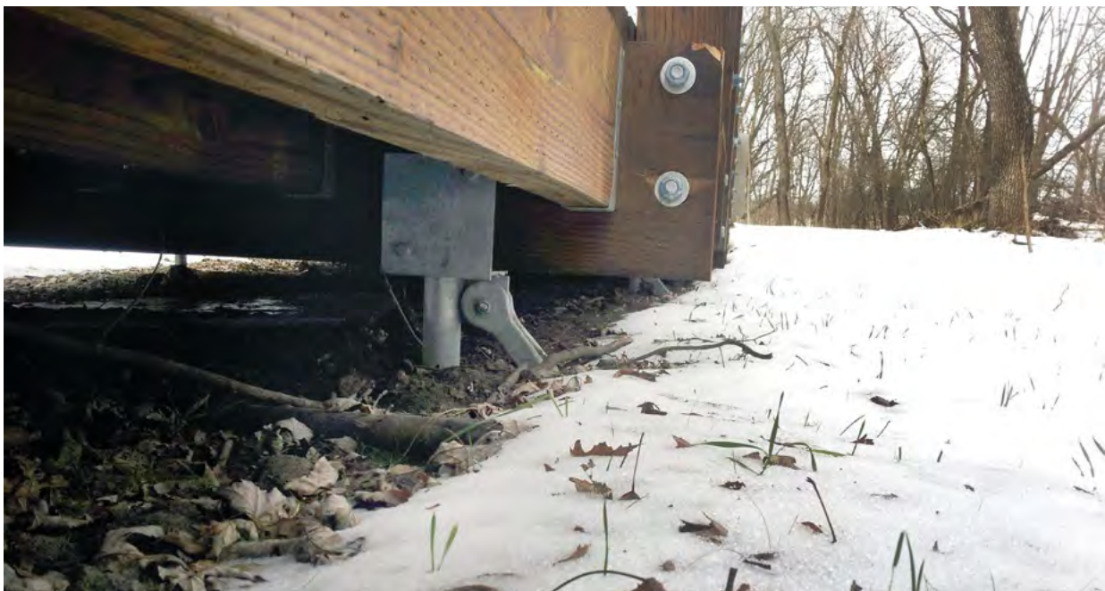
Figure 1.31 Custom saddle bracket connected with clevis to battered helical pile
