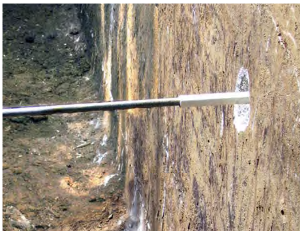
Figure 3.14 After: Shear movement recovered and wall stabilized with GeoLock anchors
