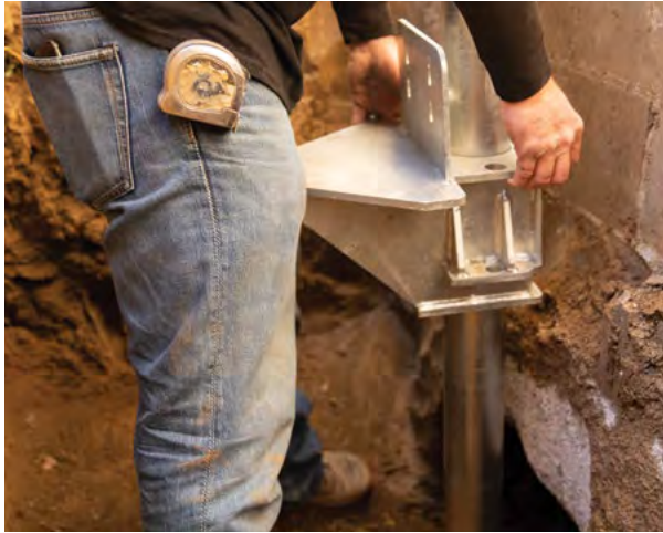
Figure 1.80 Lower assembly over pile shaft
