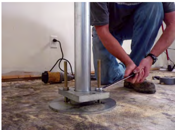
Figure 2.71 Slab pier drive adaptor installed
