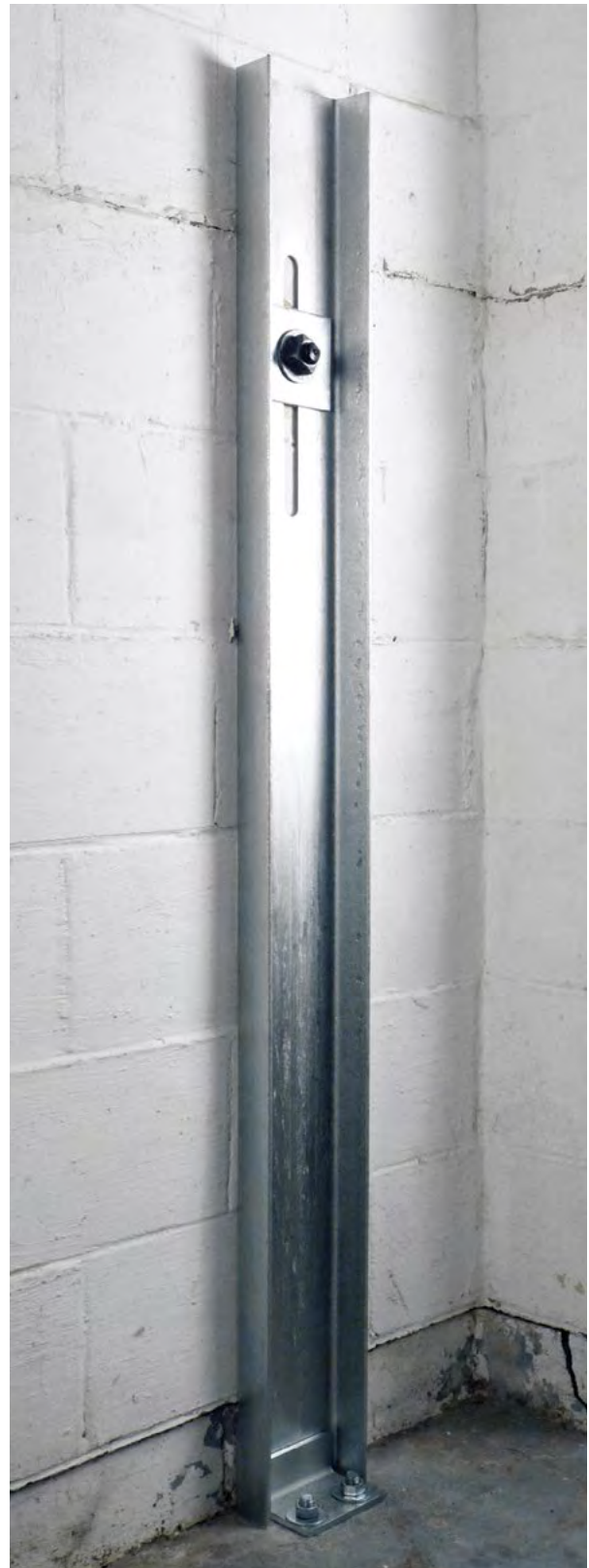
Figure 3.15 GeoLock channel anchor system installed to prevent shear movement
