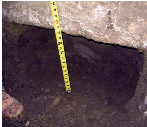
Figure 1.77 Excavation at bracket
