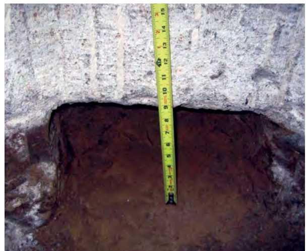
Figure 2.22 Completed footing excavation and preparation; ready to position bracket
