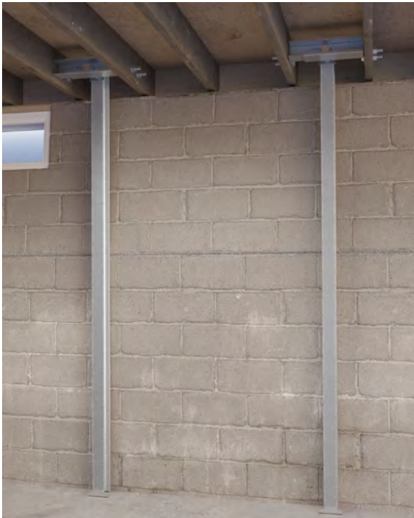
Figure 3.25 PowerBrace installation with joists perpendicular to wall
