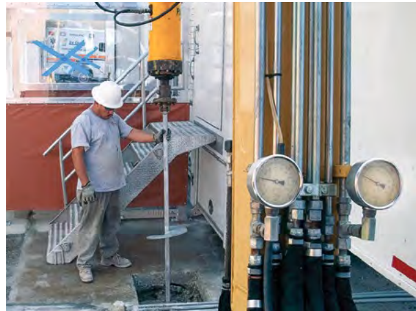
Figure 1.71 Monitoring pressure gauges while installing square shaft helical anchor
