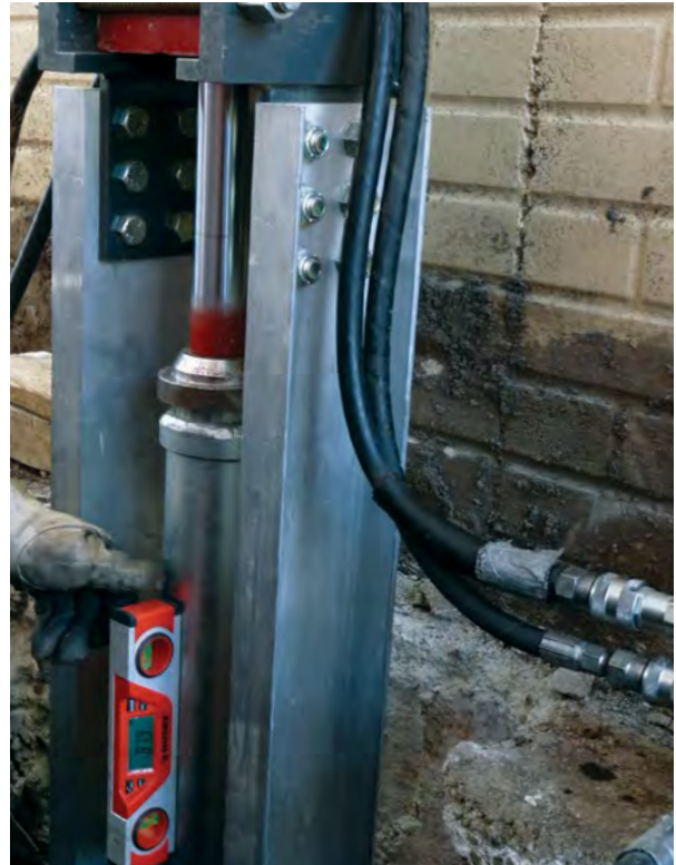
Figure 2.32 Checking drive stand alignment with digital level
