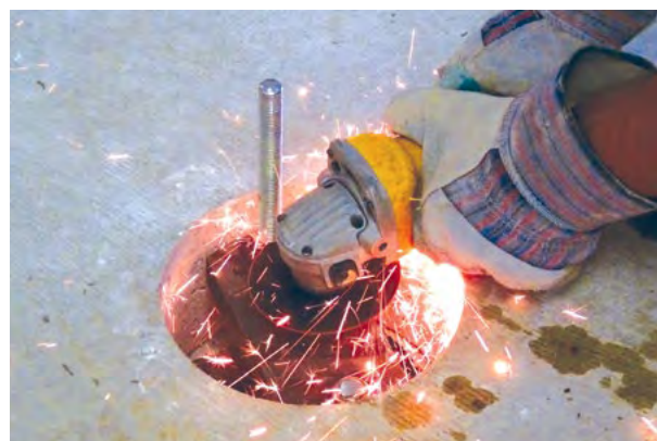
Figure 2.81 Cutting the threaded rods
