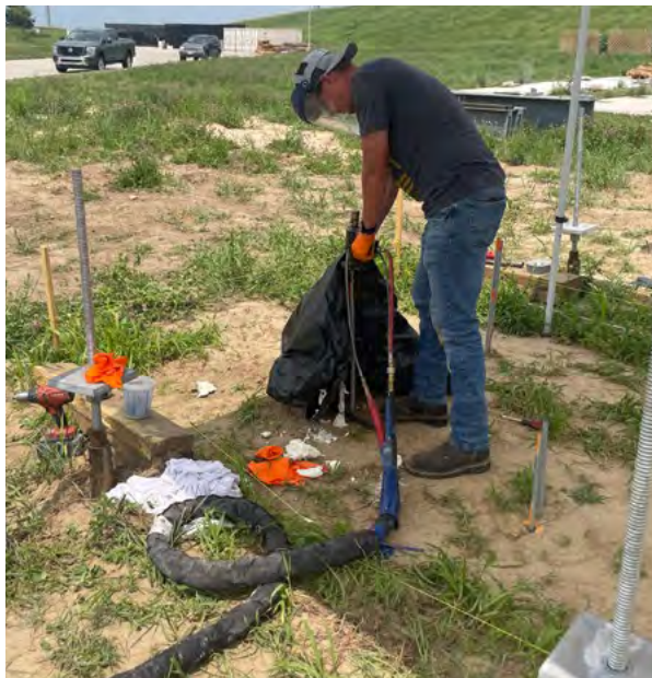
Figure 5.11 Injecting PolyLevel PLSI400H into the soil.
