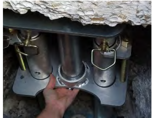
Figure 2.50 Drive stand setup within excavation
