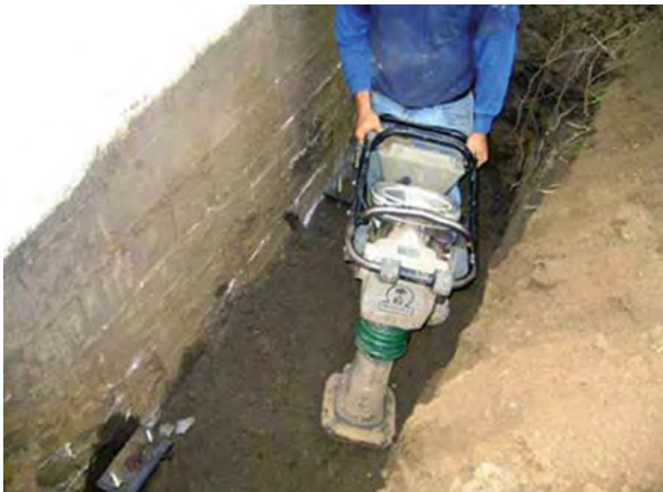
Figure 2.44 Backfill excavations and compact soil
