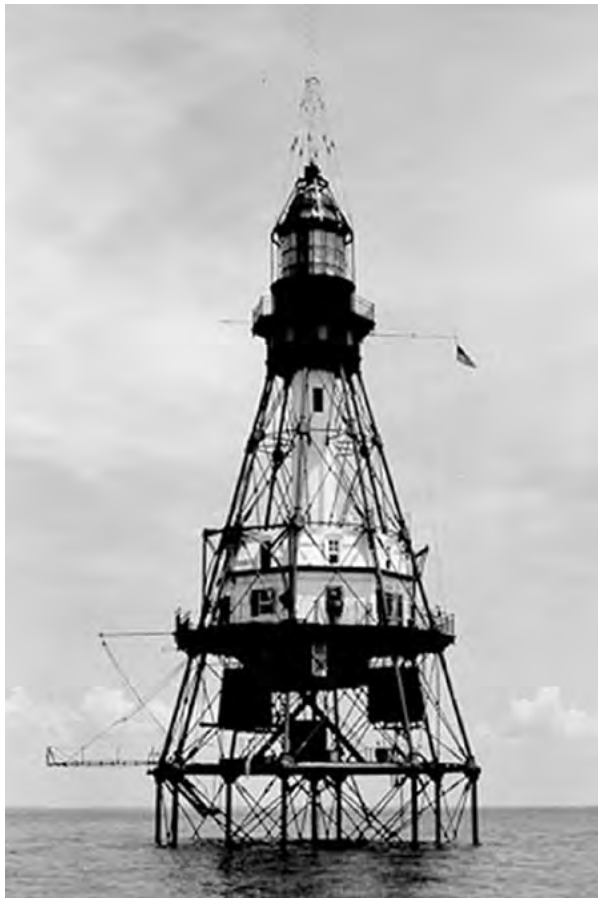
Figure 1.1 Lighthouse supported by screw (helical) pile foundations
