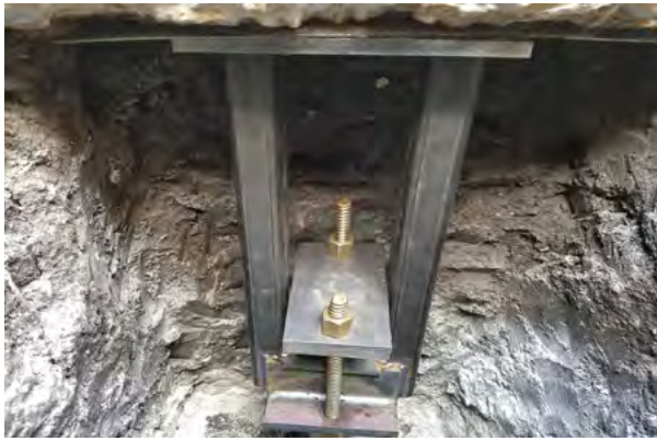
Figure 2.58 Completed concentric pier installation
