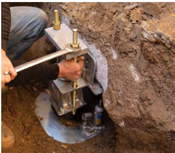
Figure 1.82 Install cap plate and rods
