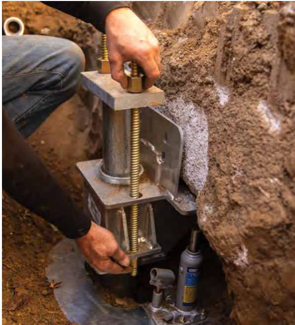
Figure 2.38 Installation of pier cap plate with coil rods and nuts
