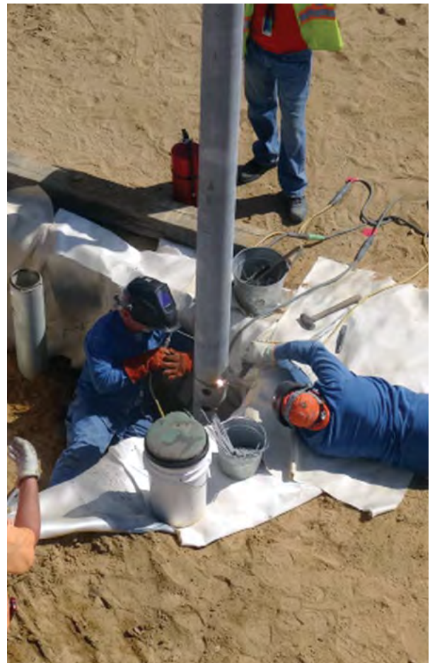
Figure 1.16 7-inch diameter pile with complete joint penetration welds between sections
