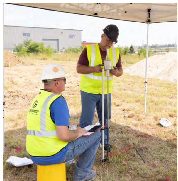
Figure 5.12 Conducting pre-injection DCP testing.
