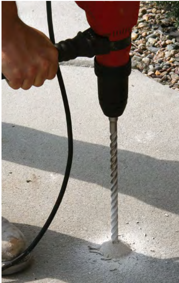
Figure 5.16 Concrete slab drilled to provide access holes
