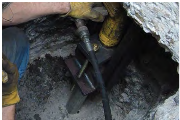
Figure 2.57 Place hydraulic cylinder and snug bracket against footing
