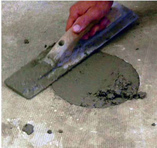
Figure 2.82 Patching holes at pier locations
