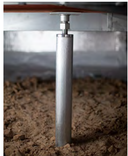
Figure 2.63 Completed Push Pier SmartJack installation. Model 288 SmartJack shown.
