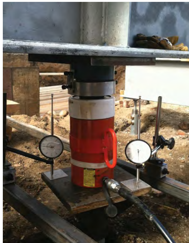
Figure 1.55 Close up of test pile, hydraulic cylinder, dial gauges and hemispherical bearing plate
