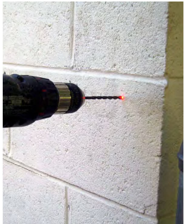
Figure 2.43 Benchmark established with a shallow hole drilled into the concrete block
