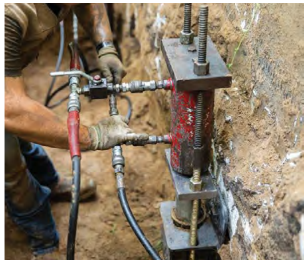
Figure 2.40 Connection of lift cylinder assembly
