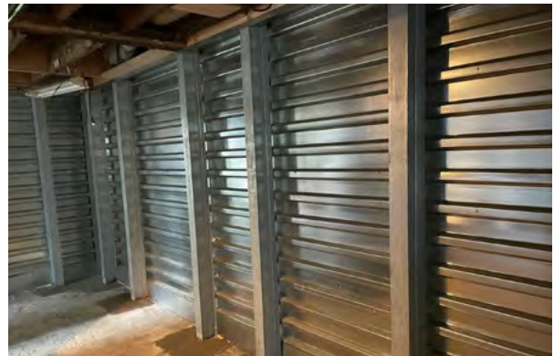
Figure 3.6 After: Wall is strengthened and permanently stabilized
