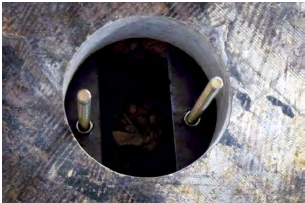
Figure 2.69 Threaded rods installed
