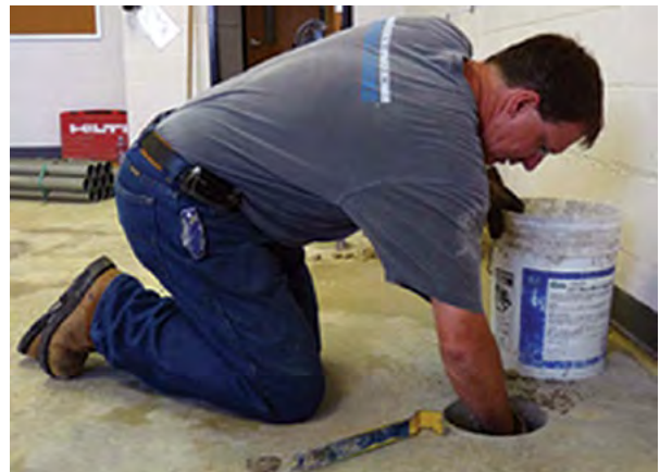
Figure 2.67 Excavating beneath the slab
