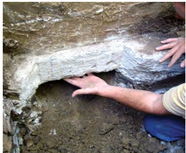
Figure 2.21 Checking underside of footing for proper preparation
