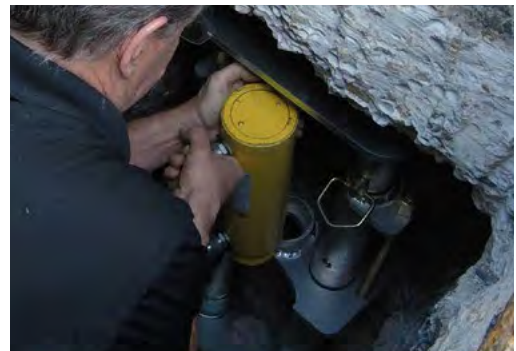
Figure 2.51 Placement of hydraulic drive cylinder
