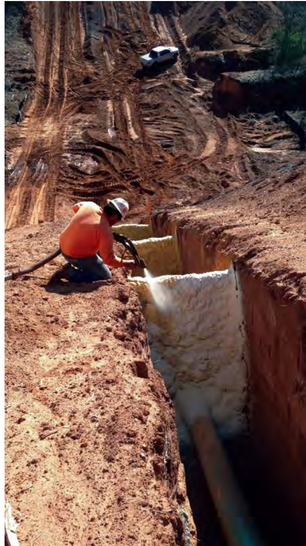
Figure 5.10 Placement of polyurethane foam trench breaks
