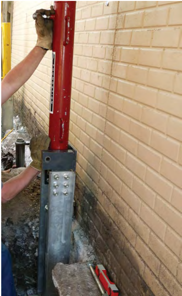
Figure 2.29 Hydraulic drive cylinder placed within top fixture of drive stand
