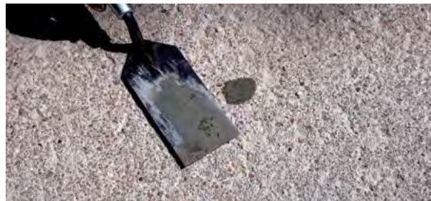
Figure 5.18 Patching the injection hole
