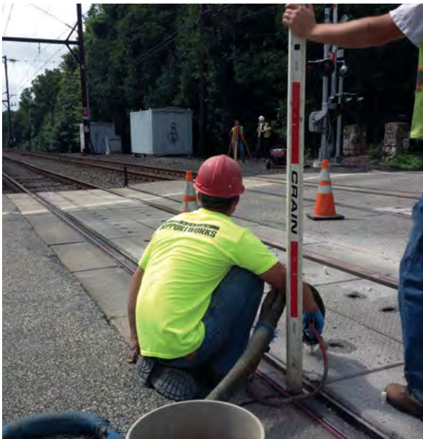
Figure 5.13 Survey equipment used to monitor rail lift from PolyLevel injection
