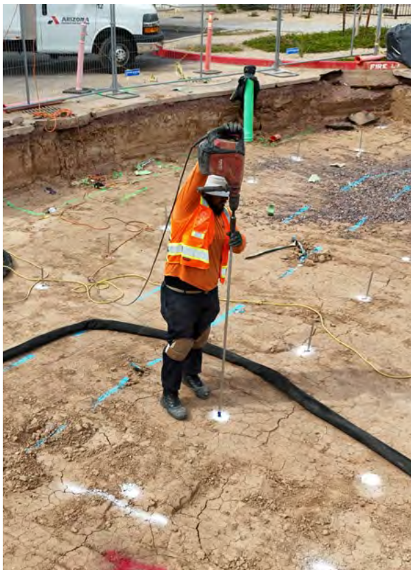
Figure 5.19 Driving injection tube
