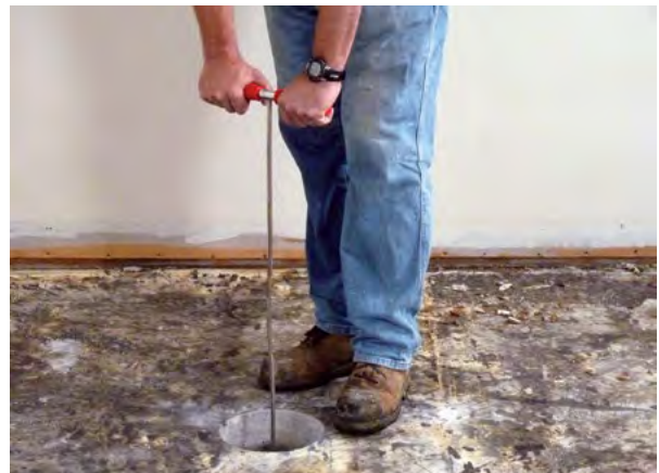
Figure 2.66 Probing for utilities or obstructions
