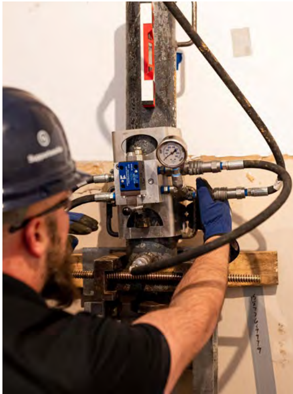
Figure 2.31 Connecting hydraulic hoses to the remote valve assembly
