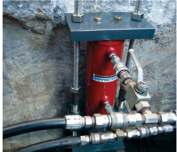
Figure 1.83 Set hydraulic lift cylinders
