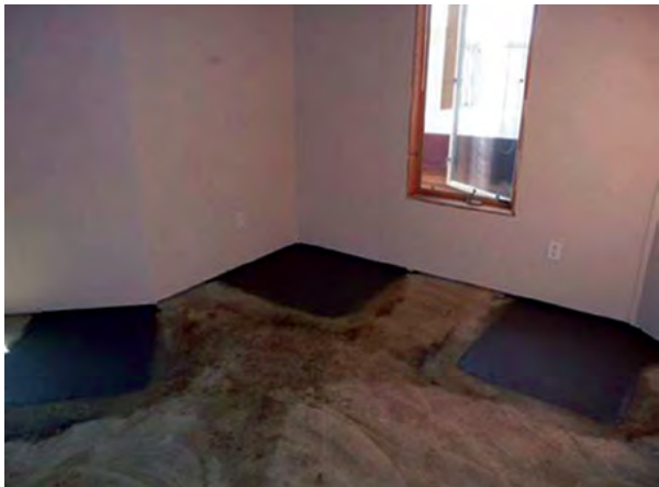
Figure 2.45 Concrete placement at interior pier locations
