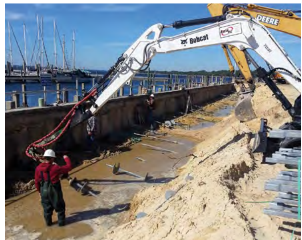
Figure 1.44 Helical tiebacks stabilize marina seawall
