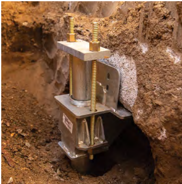
Figure 2.39 PP288 bracket ready for lift cylinder assembly
