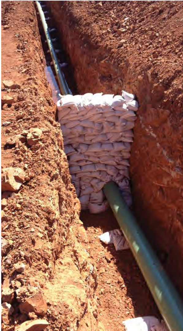
Figure 5.9 Sandbag trench breaker for pipeline
