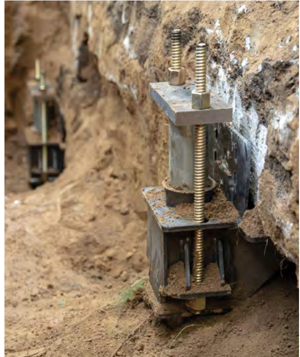
Figure 2.42 System locked off; pier installation complete
