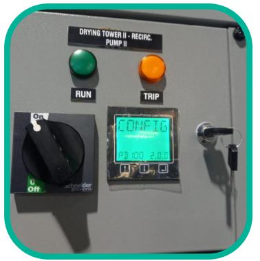
For this project, TYE received a request for the design, manufacture, and supply of thirty-six (36) motor starters with disconnectors, contactors, and overloads including 12 Process
