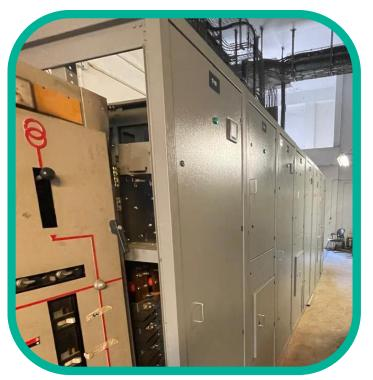
TYE's team collaborated closely with the client to deliver a solution tailored to the operational safety and redundancy requirements of the installation at a hospital in Northern Trinidad. The system was designed to manage three independent power sources via interlocked main breakers and tie-breakers, ensuring safe and reliable source selection and distribution control. The scope of works included:
