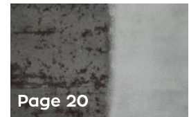
Removal of Rustgrade A
