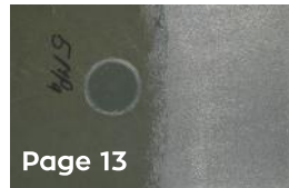
Removal of inorganic zinc primer
