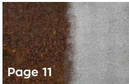
Removal of rustgrade C
