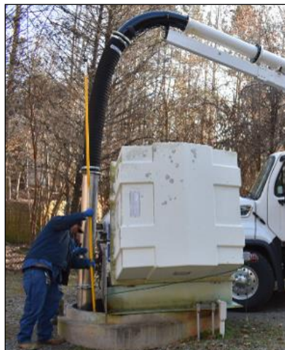
A vacuum truck (above) is used to clean out a clogged pump station. Clogs from wipes and grease can be costly to clean up and can damage equipment.
