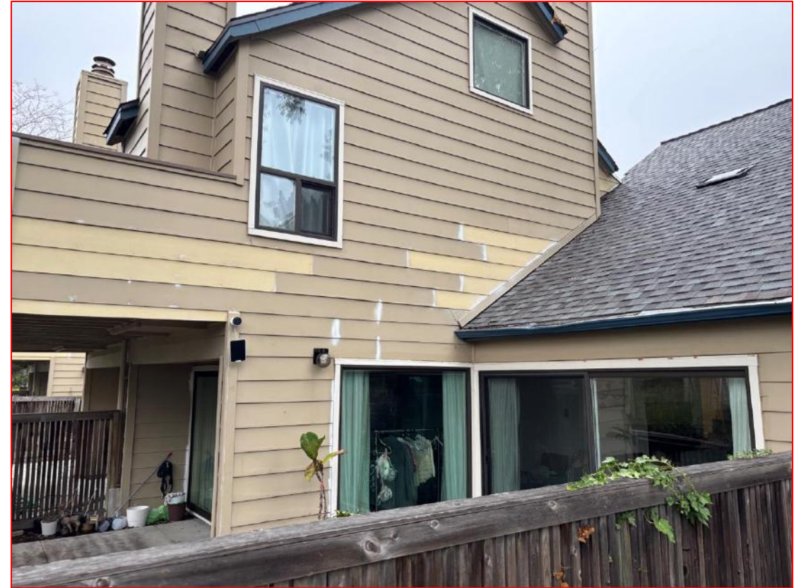
Recent "Spot" Repaired Lap Siding
