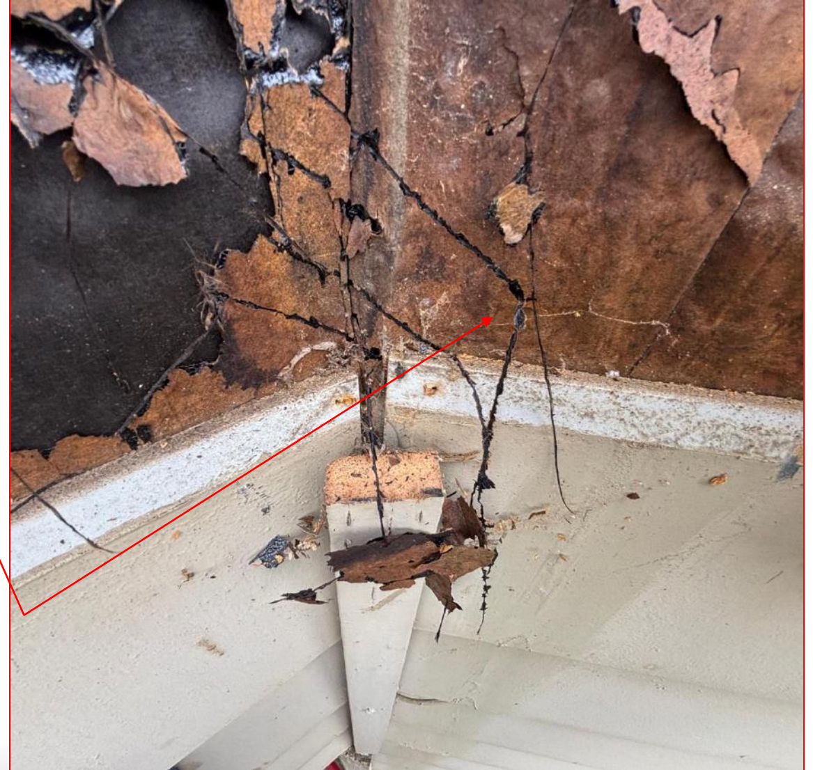
Noted Typical Felt Paper WRB System with Poly Reinforced Vertical Paper Flashing at windows, patio doors, and vertical wall transitions.
