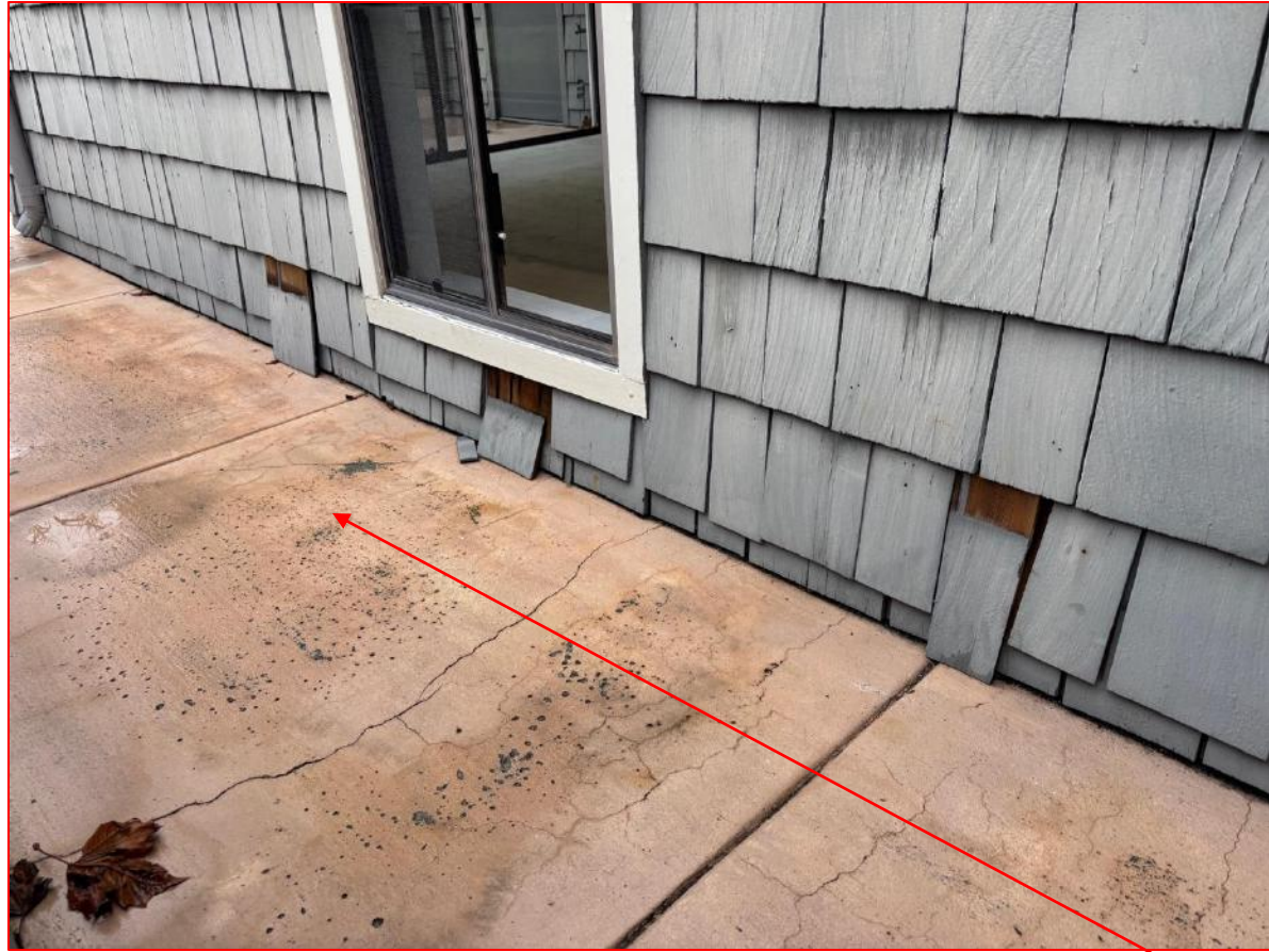
Aged, worn, and weathered balcony surface coatings. Noted varied updated ceramic tile and applied floor coatings.
