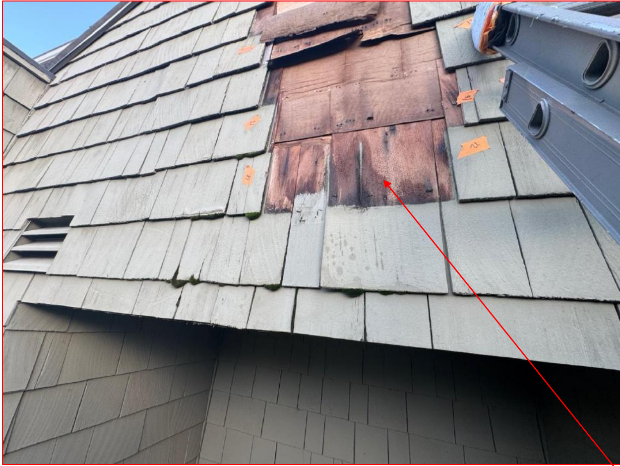
Typical Aged and Worn WRB and CDX sheathing behind painted wood shingles
