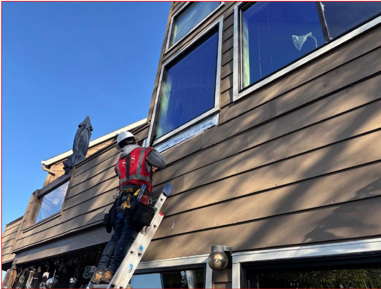
Typical Updated Flanged Window Installation, Aged WRB, and Existing Flashing Sequences. Noted Felt Paper WRB, Jamb Flashing, and Sill Flashing
