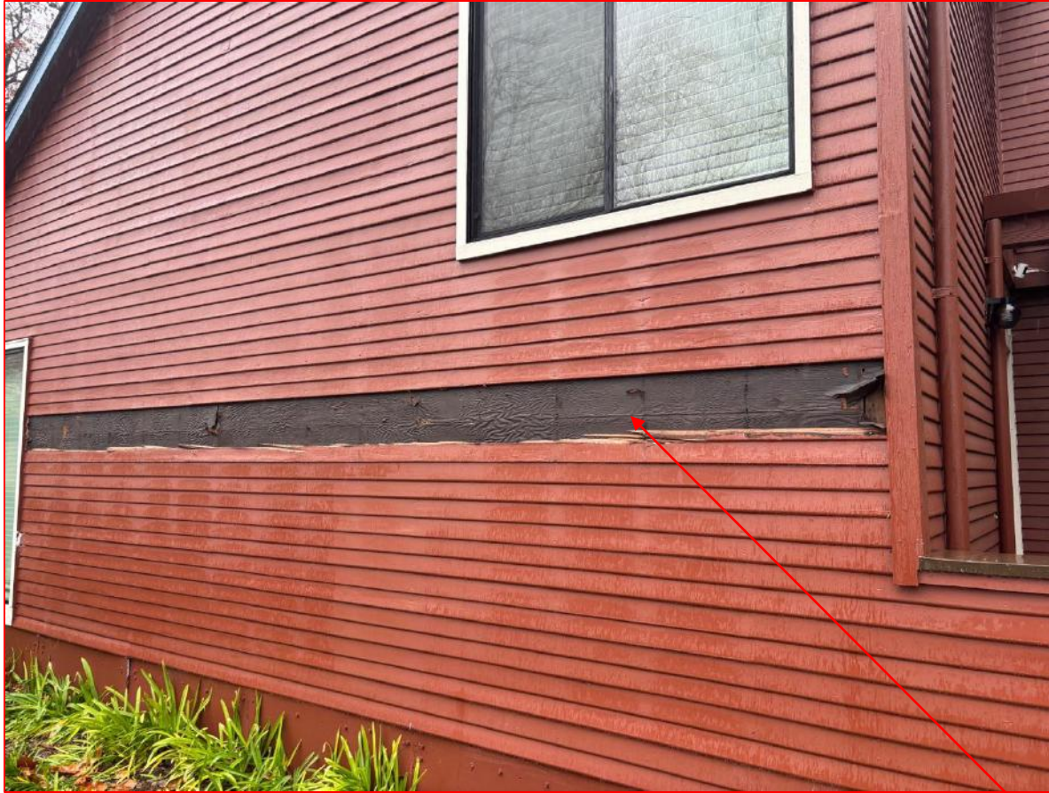
Typical Aged and Worn Felt Paper WRB behind the painted wood clapboard siding
