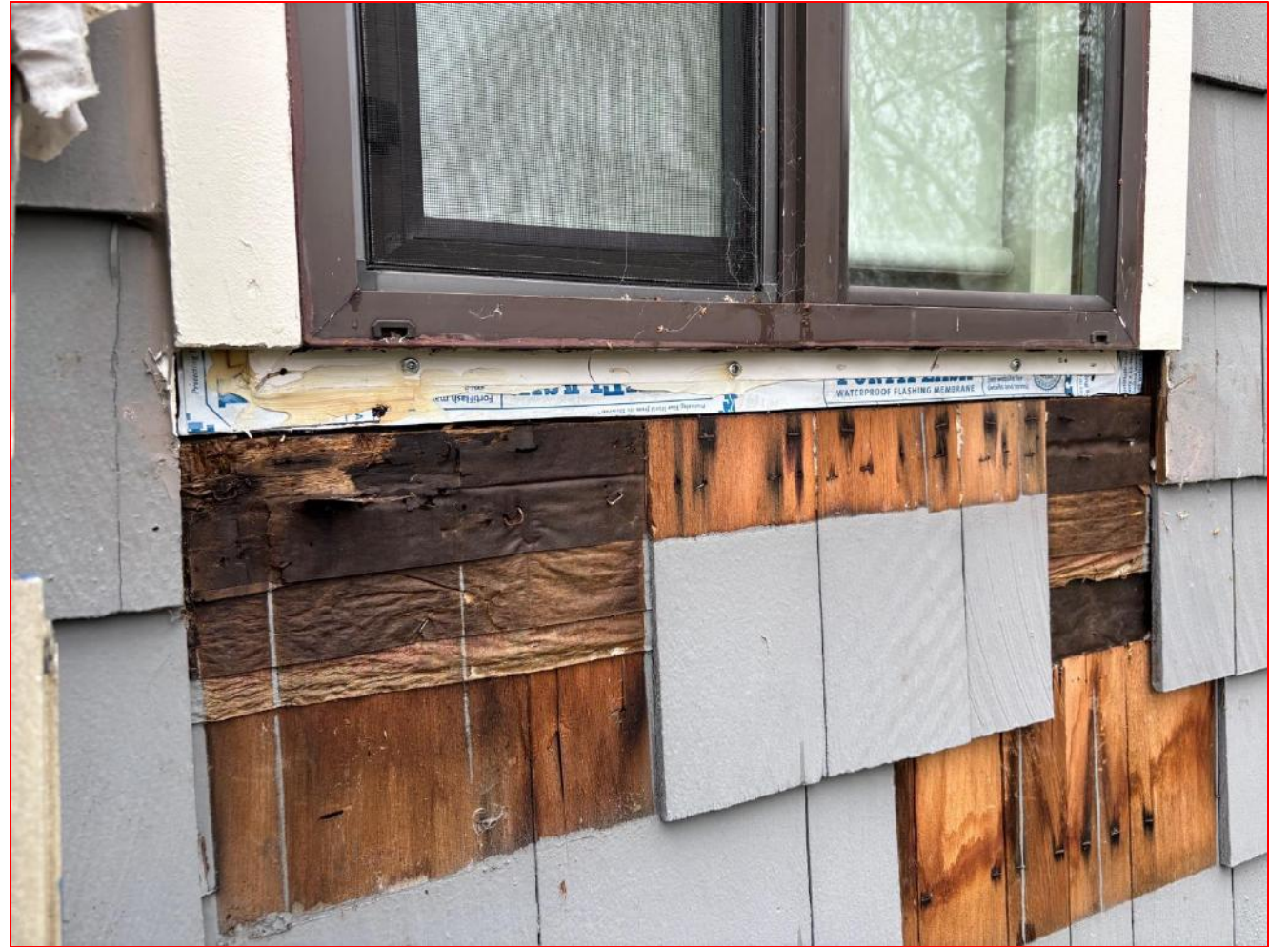
Typical Updated Flanged Window Installation, Aged WRB, and Existing Flashing Sequences. Noted Felt Paper WRB, Jamb Flashing, and Sill Flashing
