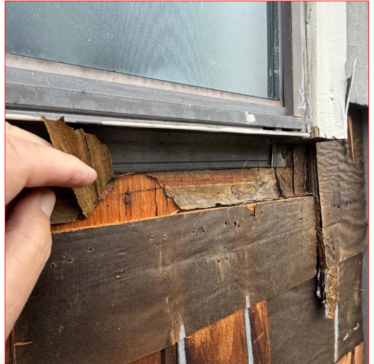
Typical Original Flanged Window Installation, Aged WRB, and Existing Flashing Sequence. Noted deteriorated window sill flashing, Felt Paper WRB, and Jamb Paper Flashing
