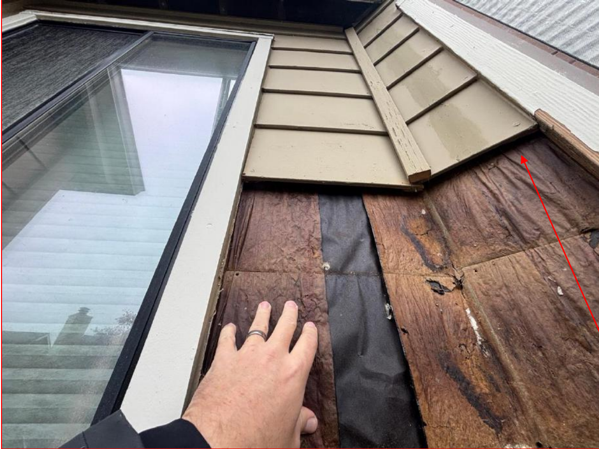
Noted Typical Felt Paper WRB System with Poly Reinforced Vertical Paper Flashing at windows, patio doors, and vertical wall transitions.
