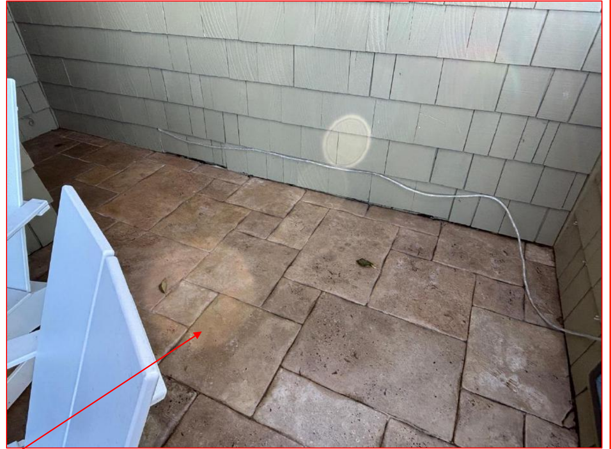
Aged, worn, and weathered balcony surface coatings. Noted varied updated ceramic tile and applied floor coatings.
