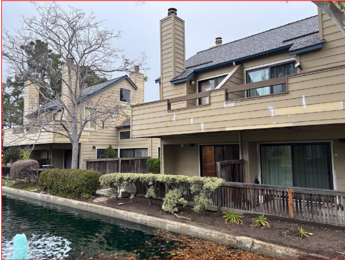
Recent "Spot" Repaired Lap Siding
