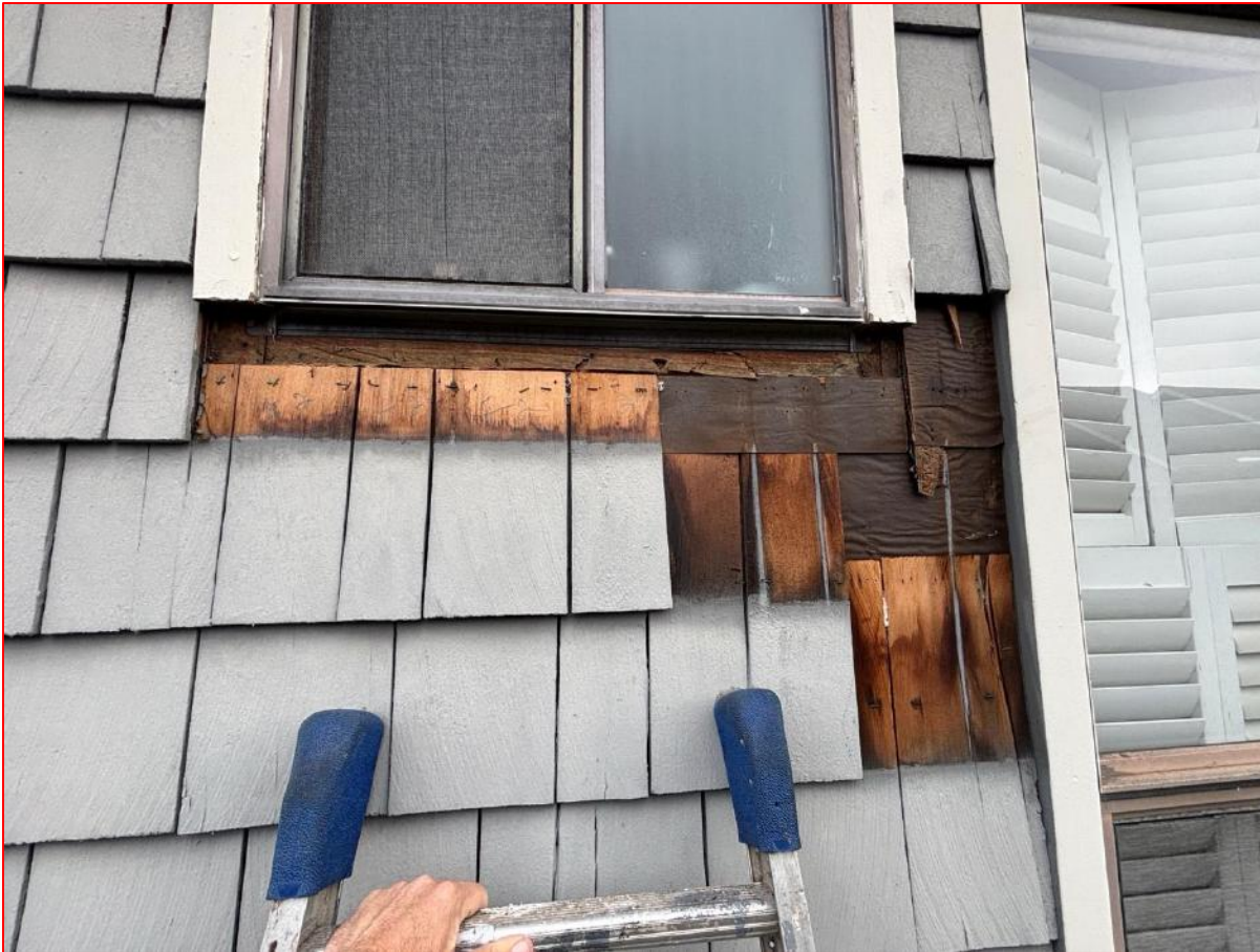
Typical Original Flanged Window Installation, Aged WRB, and Existing Flashing Sequence. Noted deteriorated window sill flashing, Felt Paper WRB, and Jamb Paper Flashing
