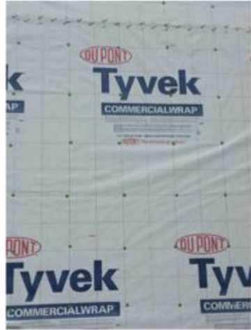
IMAGE OF TYVEK COMMERCIAL WRAP INSTALL AND FASTENING PATTERN
