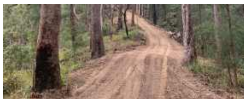
Springbrook NP fire trail after restoration - supplied
