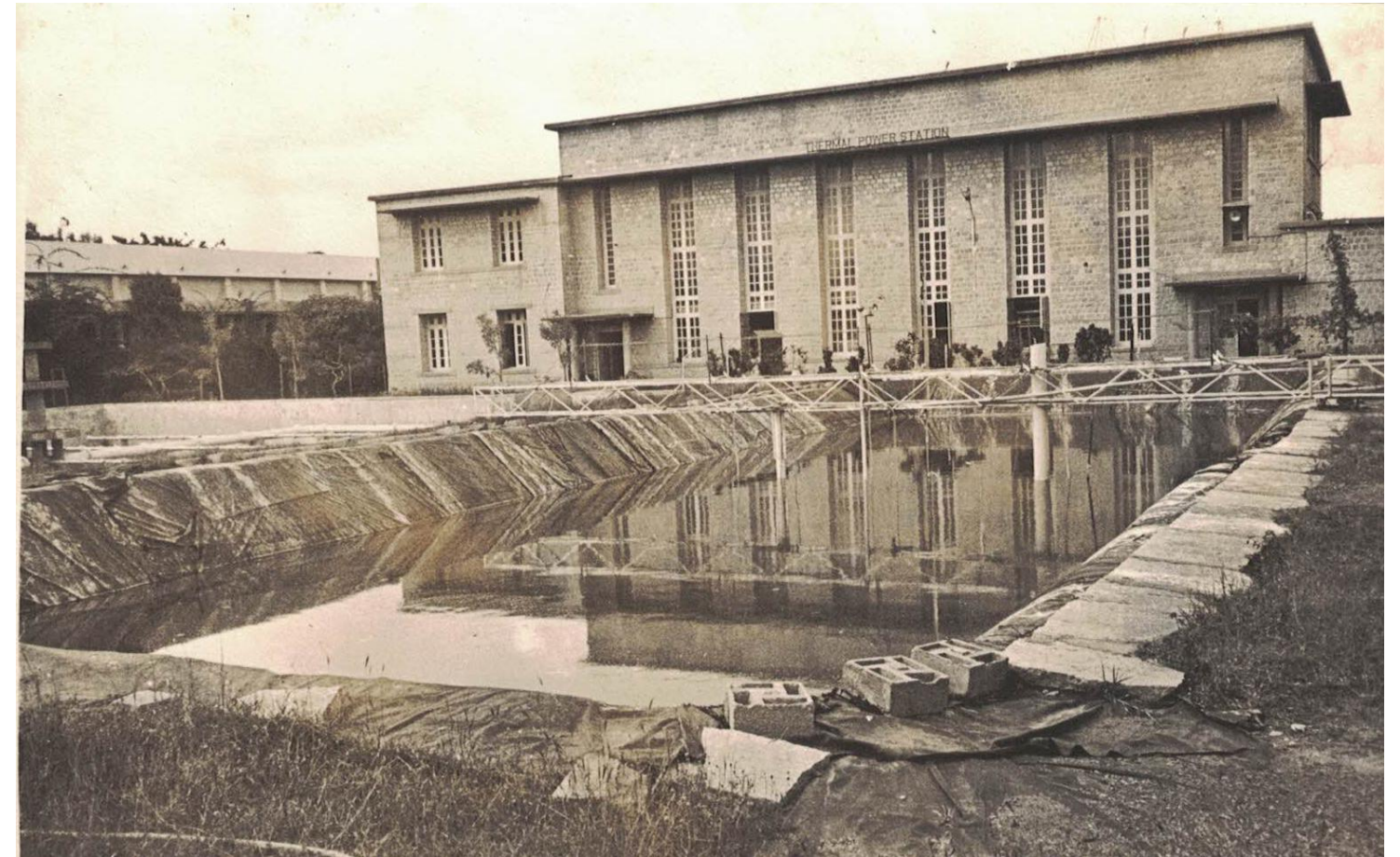
A hot ticket: The solar pond in front of the TPS building
