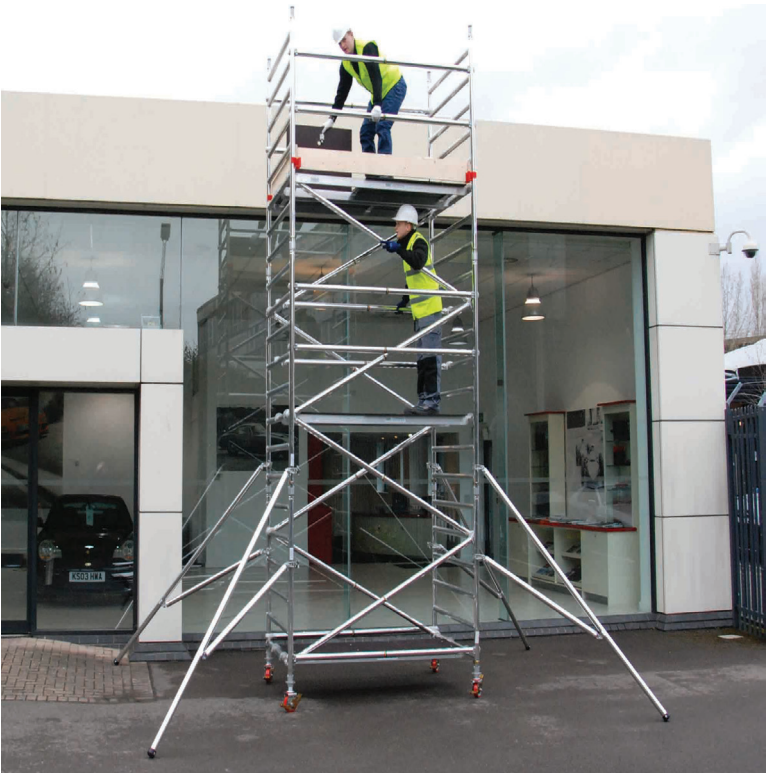
Double width scaffold tower with 3T compliant construction.
