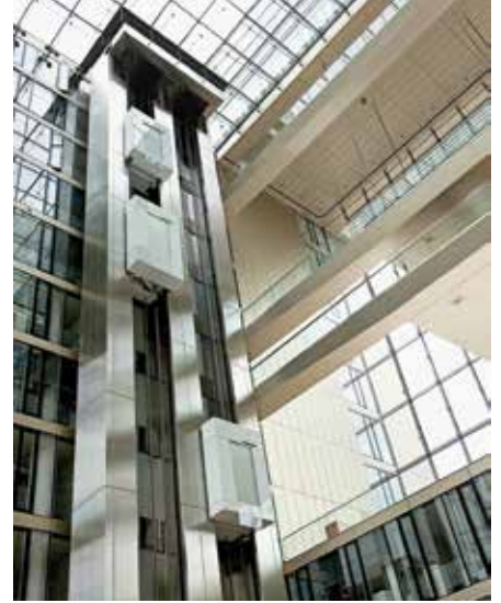
TWIN, TK Elevator's dual-passenger system in a single shaft
