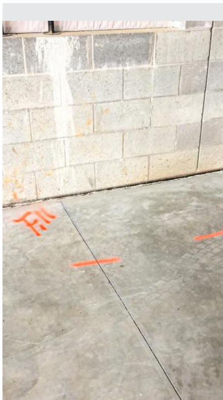
On another Welch Tile project, the tile contractor used a 10' straightedge to identify high and low spots that need additional substrate prep work.
