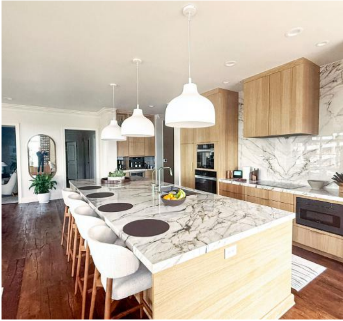
Parsons and his team have a reputation for making porcelain countertops when others say ‘no.’ This kitchen in a downtown Raleigh condo used Neolith 12mm slabs for a 16’-long island and book-matched full-height backsplash. The project was the last kitchen made before switching over to the company’s new CNC machinery.
