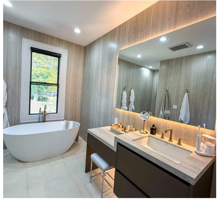
Parsons and his team had to execute floors, walls, and countertops in this North Carolina mountain home during a blizzard, using 6mm and 12mm porcelain slab materials.
