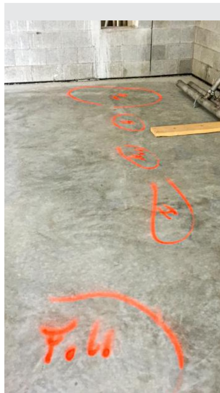
On another Welch Tile project, the tile contractor used a 10' straightedge to identify high and low spots that need additional substrate prep work.
