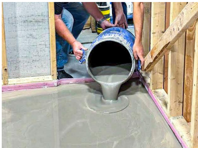
At another NTCA Regional Training program, self-leveling compound is poured to attain floor flatness
