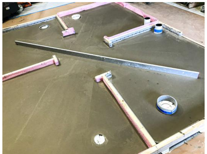
At a 2021 NTCA Regional Training program held at D.W. Sanders Tile & Stone Contracting, a 10' straightedge is used on a flat floor achieved by a self-leveler.
