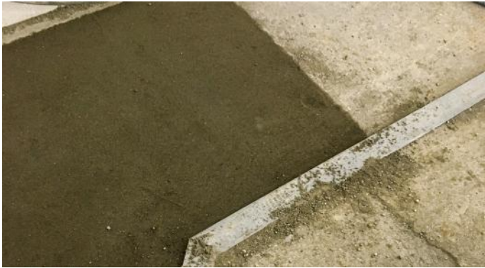
Installers at Welch Tile used a mortar bed to achieve the desired floor flatness.
