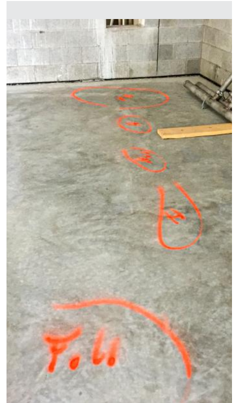
On another Welch Tile project, the tile contractor used a 10' straightedge to identify high and low spots that need additional substrate prep work.
