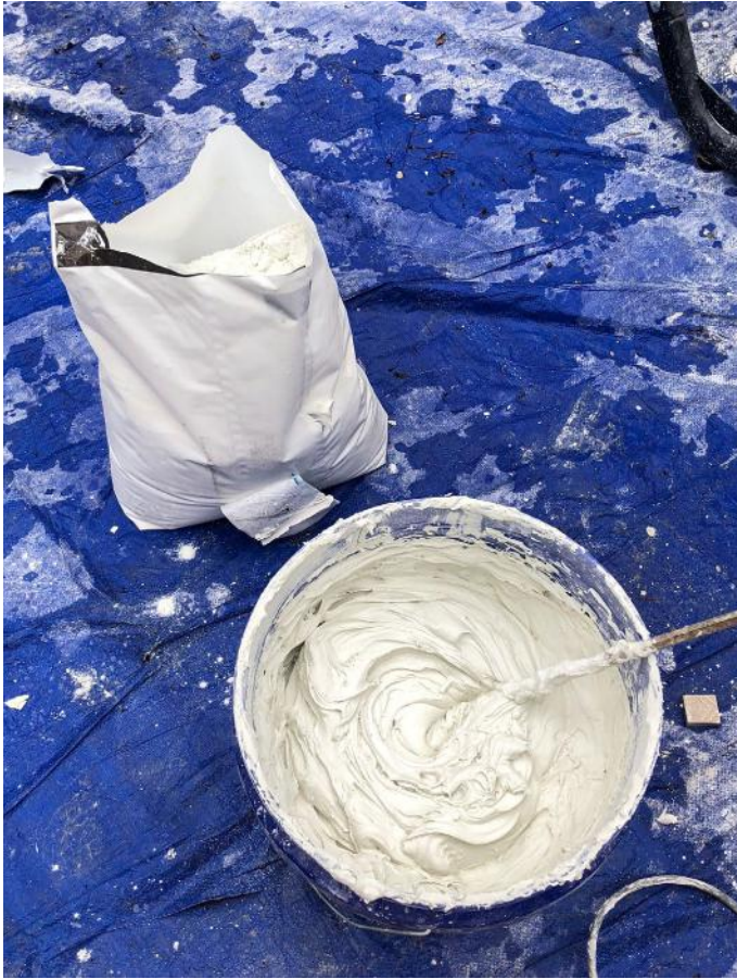
Mixing is one of the first steps in the installation process, and it sets the stage for everything that follows. Follow the mortar manufacturer's mixing speed instructions!
