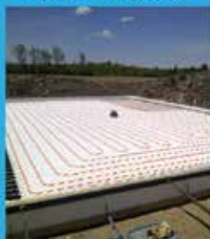
Hydronic Floor Heating
