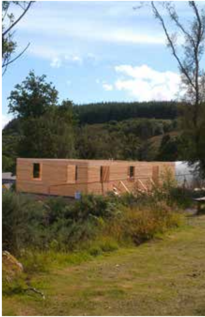
- Half built walls
