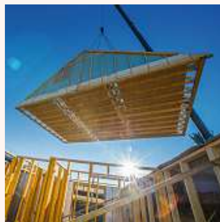
Above Pre-fabricated trussed rafter roof and spandrel panel construction being lifted into position.
