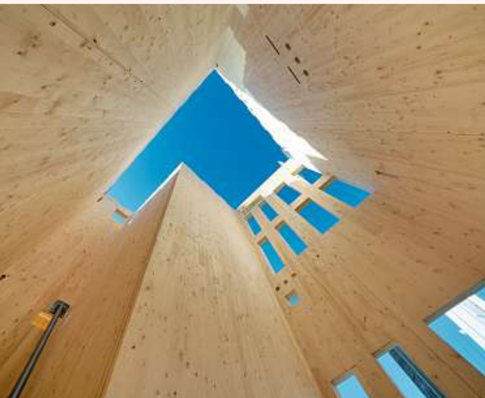
Above Cross-laminated timber structure during construction.
