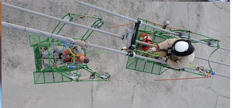
ABOVE Los Angeles Department of Water & Power tower transmission linemen use an AZTEK jigger to rescue another linemen in a line cart off the conductor mid span. Line carts as shown are used for placing spacers on multiple conductors and for doing repairs mid span on power lines. LEFT: Waldo Etherington, an adrenaline “junkie”, lowers out of a hot air balloon in Dorset, UK at 1,000’ off the ground on an AZTEK SOF with the other end as a safety. No helmet, but of course, what would a helmet do for him?
