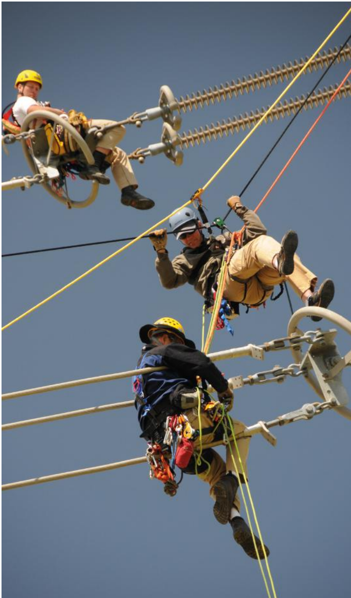
ABOVE: RTR instructor, Keith Thorne (top), watches a pick off of a firefighter 'casualty' from a power transmission line using an AZTEK from a rescuer using a tracking line offset. Photo from RTR Offset Highline Rescue Workshop at Western Area Power Admin. At Elevelta, California 2017.
