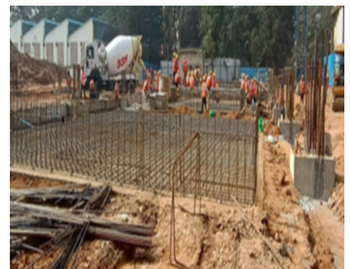
FEBRUARY 2 (DAY 2): GRADE SLAB CONCRETING
