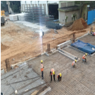
FEBRUARY 1ST (DAY 1) GRADE SLAB REINFORCEMENT
