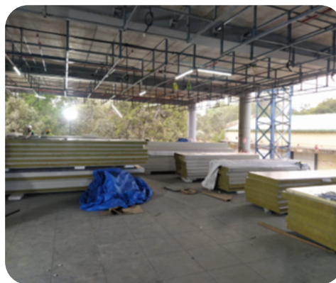
FEBRUARY 8 & 9 (DAY 8 & 9): INTERIOR WALL PANELS AND OTHER INTERIOR ELEMENTS STACKED.
