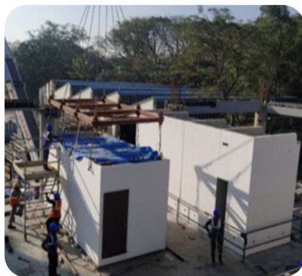
FEBRUARY 7 (DAY 7): POSITIONING OF PREFABRICATED PREFINISHED TOILET PODS
