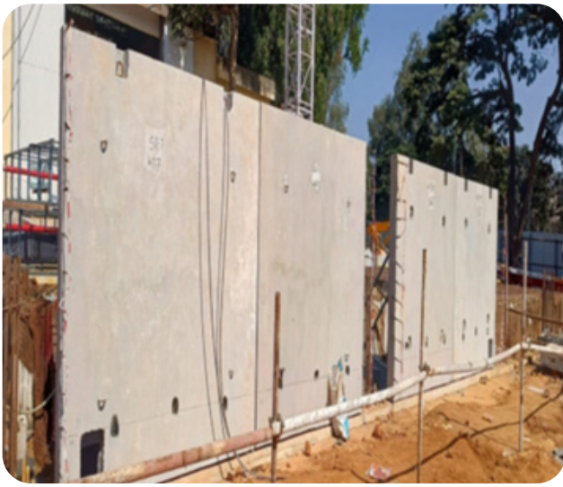
FEBRUARY 3 (DAY 3): 2D PRECAST RC WALLS ON GF
