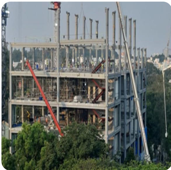
FEBRUARY 23 & 24: FIFTH FLOOR BEAMS & SLABS ERECTED.
