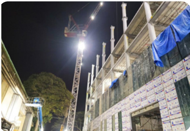
FEBRUARY 20 & 21: UNITIZED STRUCTURAL GLAZING SYSTEM INSTALLATION AT GROUND FLOOR AND FIRST FLOOR
