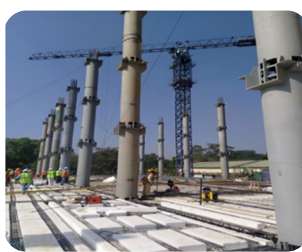
FEBRUARY 12 & 13: STRUCTURAL COLUMN SPLICE AT SECOND FLOOR LEVEL
