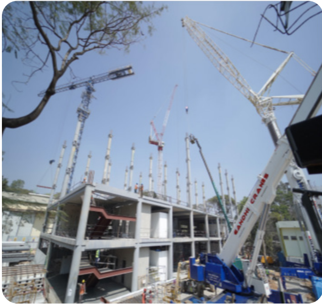
FEBRUARY 14 & 15: SECOND TO FOURTH FLOOR COLUMNS ERECTED
