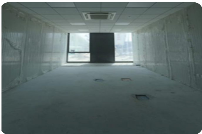
February 28: Prefinished modular walls are installed in the first floor on false flooring system.
