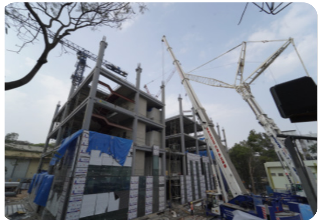
FEBRUARY 22: FOURTH FLOOR STRUCTURAL ELEMENTS ERECTED.
