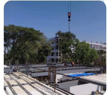
FEBRUARY 6 (DAY 6): BEAMS ERECTION
