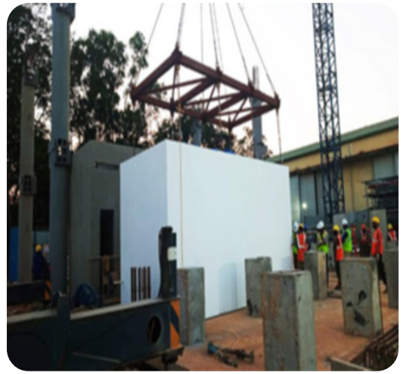
FEBRUARY 4 (DAY 4): PREFABRICATED PREFINISHED TOILET PODS PLACED IN POSITION ON GF
