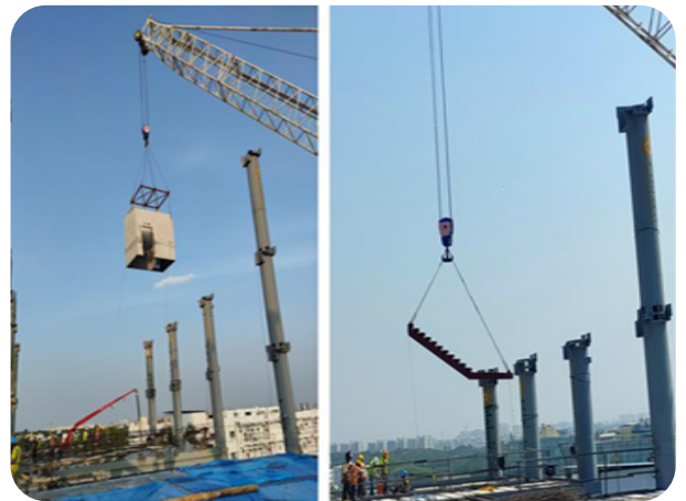
FEBRUARY 19: PREFABRICATED PREFINISHED LIFT PODS & PREFABRICATED STAIR CASE ERECTED.
