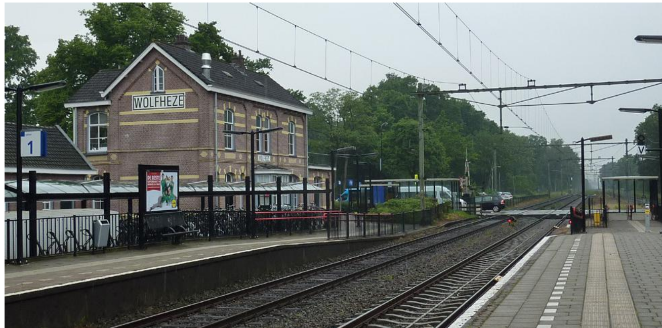
Emplacement van station Wolfheze.
