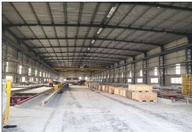
Figure 3: IN-Site Casting Yard for Precast
