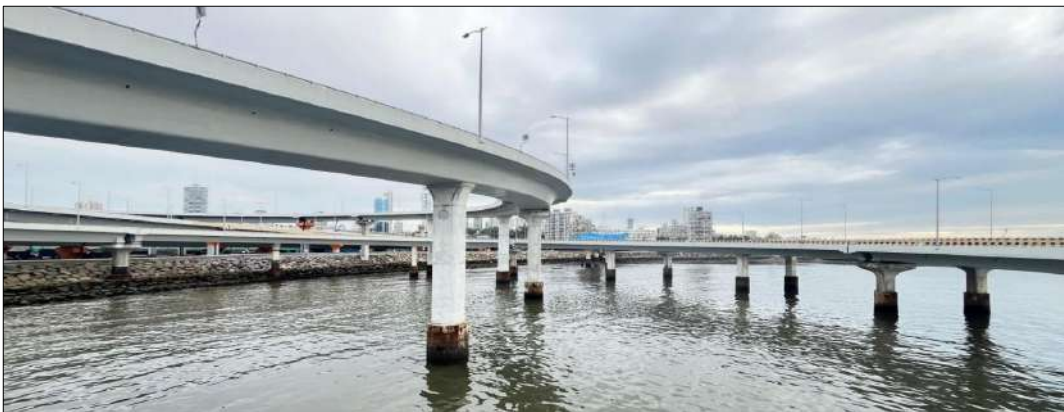
Figure 8: Bridge Deck with Monopile (Actual Picture)
