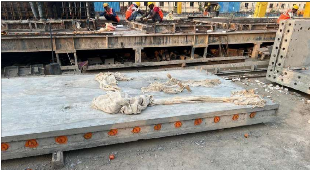
Figure 5: Precast Slab from Site Visit
