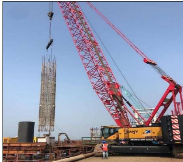
Figure 6: Rebar Cage Installation
