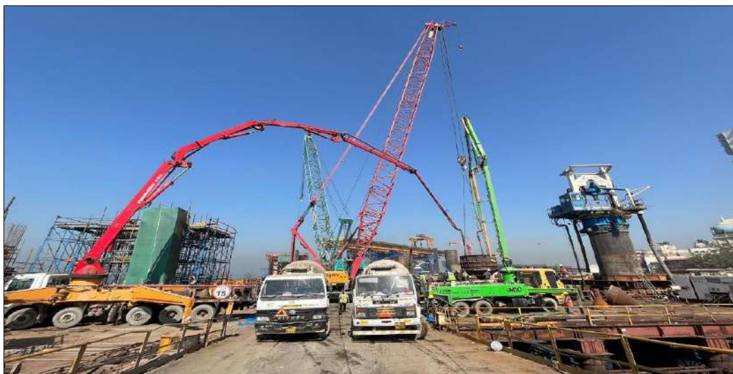
Figure 7: Concrete Pour with Two Placer Booms
