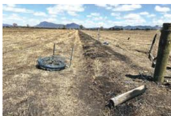
Preparing to run out multiple wire strands
