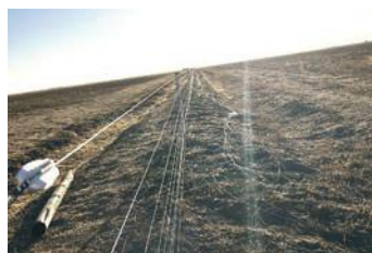
Wire strands tensioned and clipped
