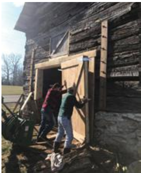
Bobby and Mike putting up doors on the old stable.
