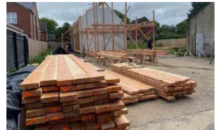
- Wood planed on the Logosol 4-sided planers, ready and waiting in perfect dimensions to be made into a timber-frame house by Groscope, a social housing project in Hull that provides affordable housing for homeless and vulnerable people. It also helps them to learn skills by encouraging them to be involved in the building/renovating process.
