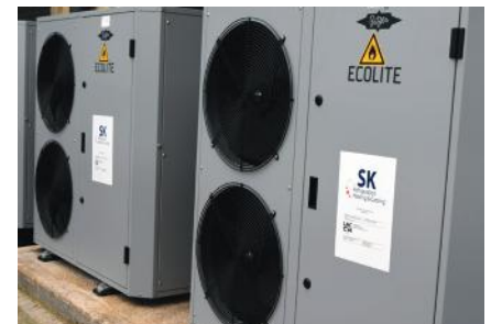
The BITZER ECOLITE condensing units operate on low-GWP R454C refrigerant
