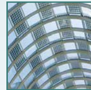
Glass Integrated PhotoVoltaics (GIPV) to harness solar energy
