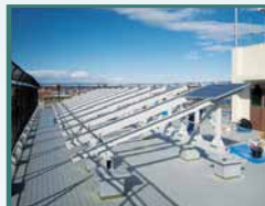
Fibre Reinforced Plastics (FRP) to create light-weight and durable structures
