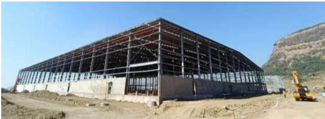
Figure 2: External View of the PEB Structure
