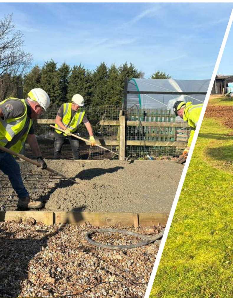
During and after the renovation work
