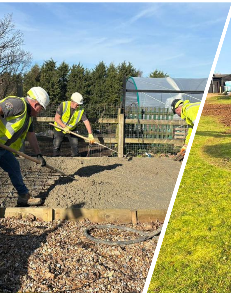
During and after the renovation work
