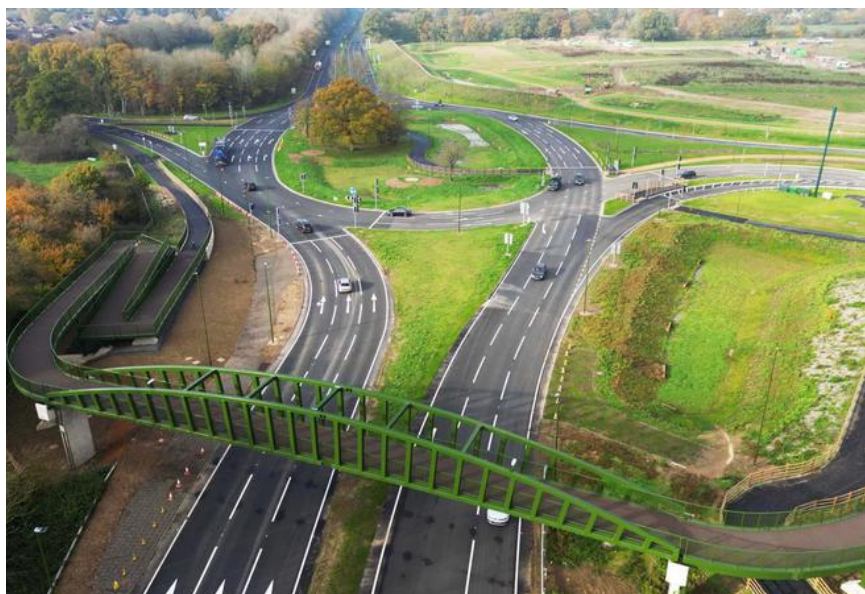
52-metre Vierendeel-Style Footbridge
