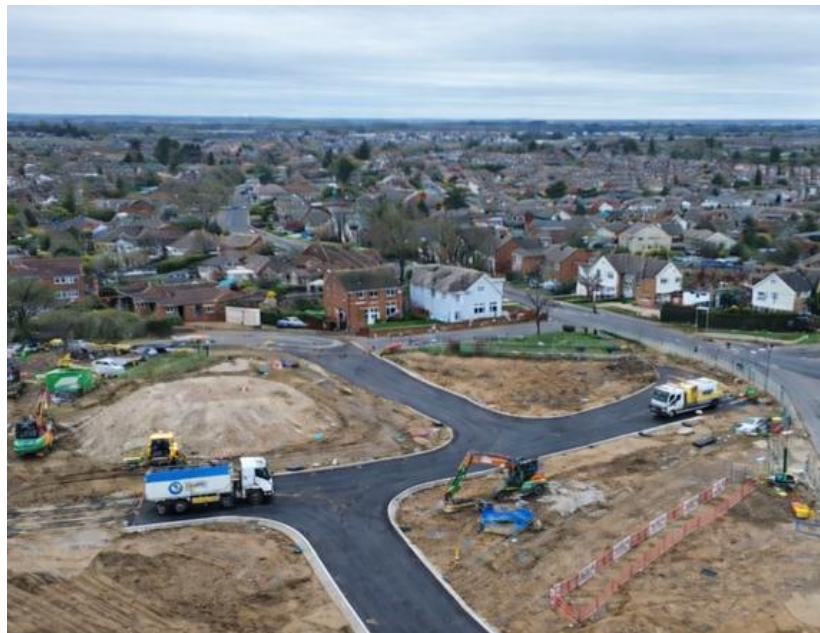
March Progress Photo from our Stanway Project
