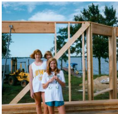
SUMMER 1992 Sheré, Natalie, and Emily during a visit during the construction
