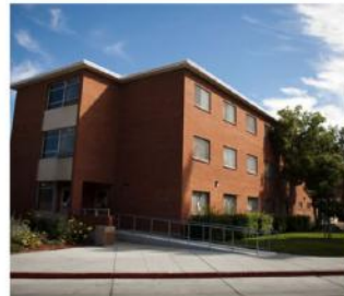
CV3 Project: Replace Washburn, Joe West and Dining Commons for a net addition of 1,000 beds and new dining facility over phases.
