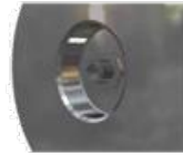
Counterbored recess for M12 connector fitting
