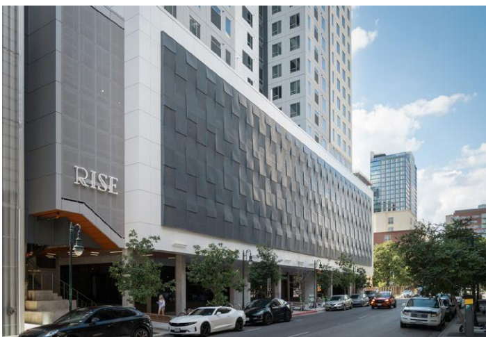
RISE AT WEST CAMPUS AUSTIN, TEXAS
