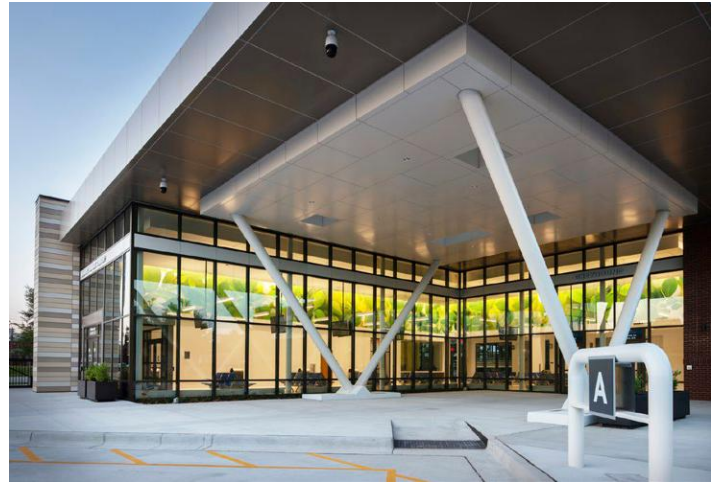
ALBANY TRANSPORTATION CENTER ALBANY, GEORGIA
