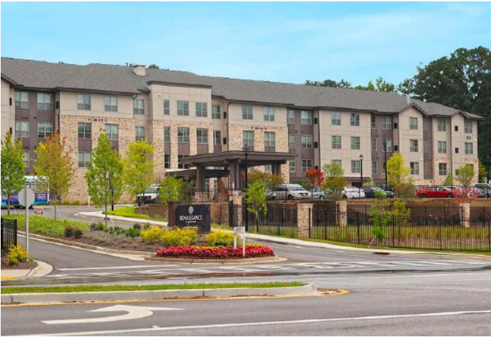
RENAISSANCE AT GARDEN WALK RIVERDALE, GEORGIA
