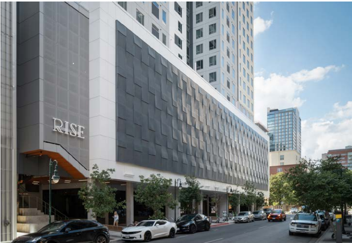
RISE AT WEST CAMPUS AUSTIN, TEXAS
