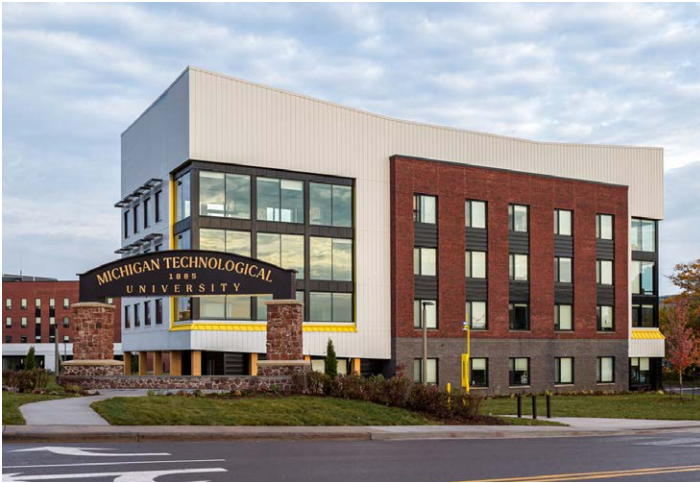
MICHIGAN TECH, EAST HALL HOUGHTON, MICHIGAN
