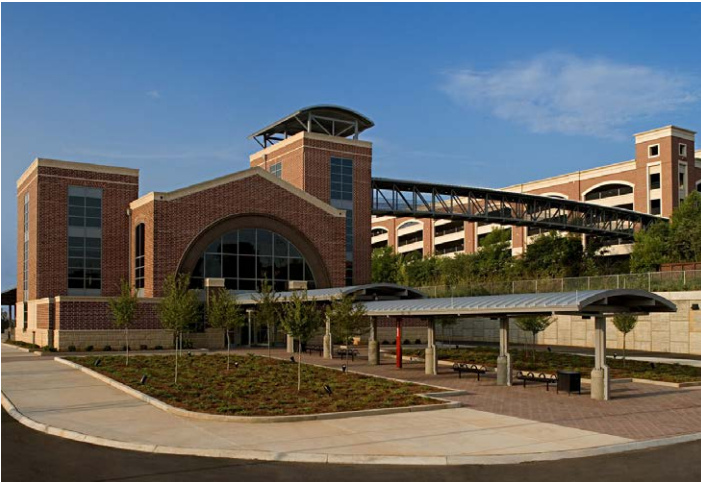
ATHENS MULTIMODAL TRANSIT CENTER ATHENS, GEORGIA
