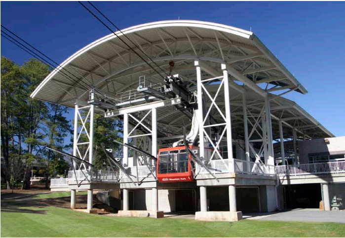
STONE MOUNTAIN AERIAL TRAM STATION STONE MOUNTAIN, GEORGIA
