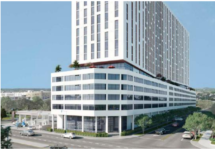
CASA AT FIU SWEETWATER, FLORIDA
