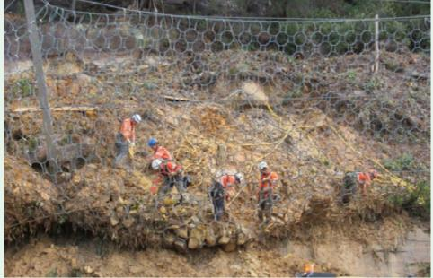
To prevent potential damage to trains and infrastructure, Shahram designed a five-meter high rockfall barrier capable of supporting 3,000 kilograms of fallen rocks. Shahram worked closely with installation teams from Major Works and Safety Environment Quality Risk and the barrier was completed in June 2021.
