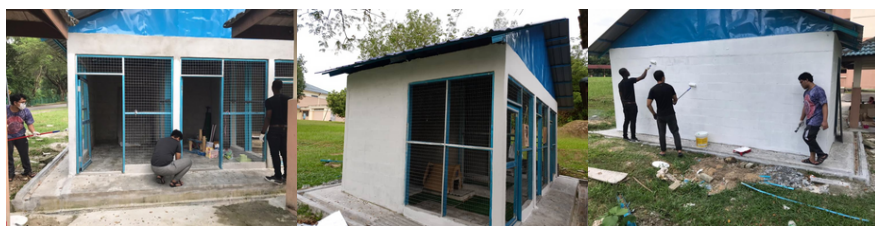
Construction of the cat shelter
