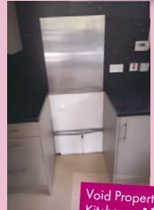
Void Property – Kitchen – Before
