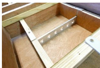
Fig 9 Mounting the Earth Bar
