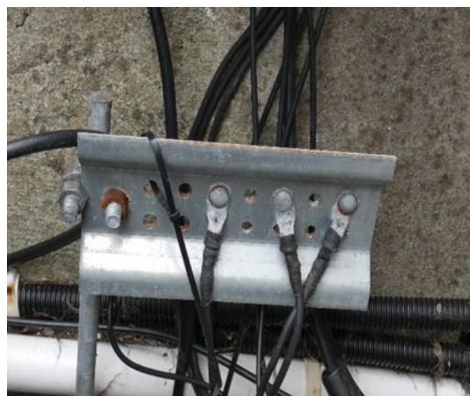
Fig 12 three cables connected to Earth Rod
