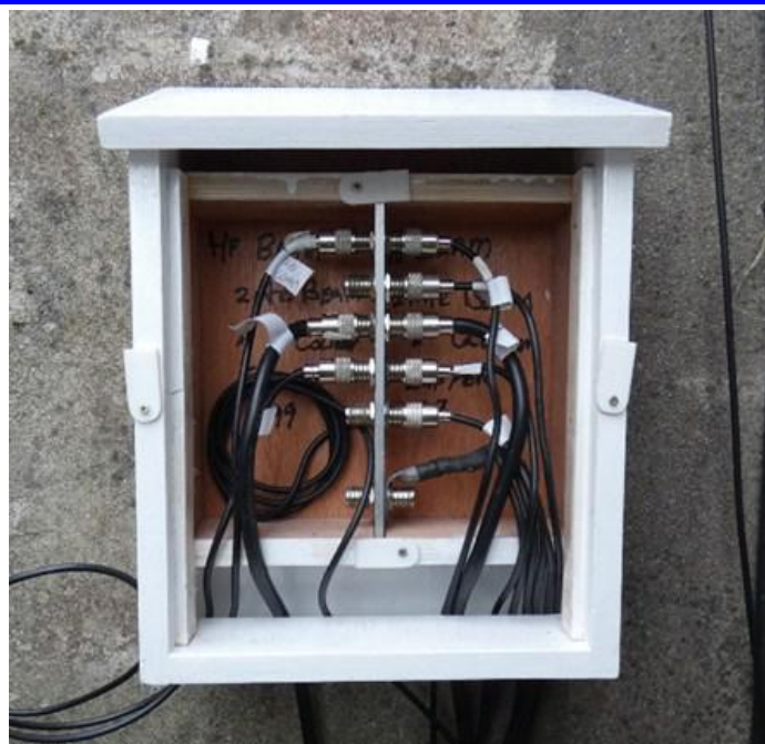
Fig 11 Box in place with cables from the house connected to the antenna coax cables
