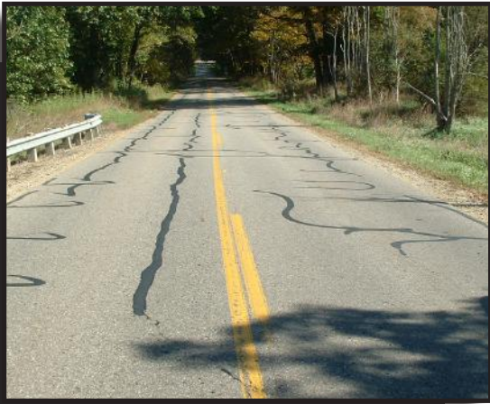
Crack seal on O Avenue
