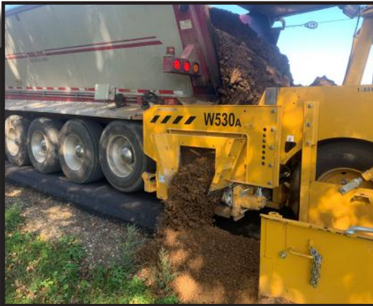
Placing shoulder gravel on XY Avenue
