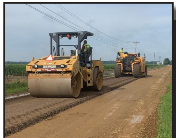
Pulverizing XY Avenue
