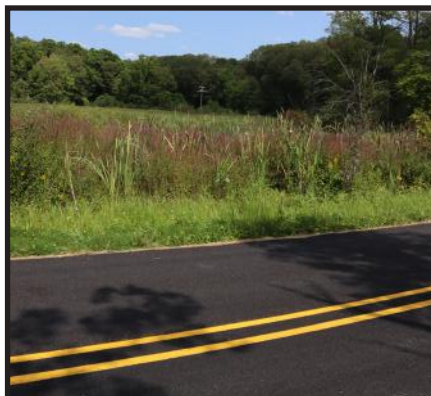
Chip seal/fog seal on EF Avenue
