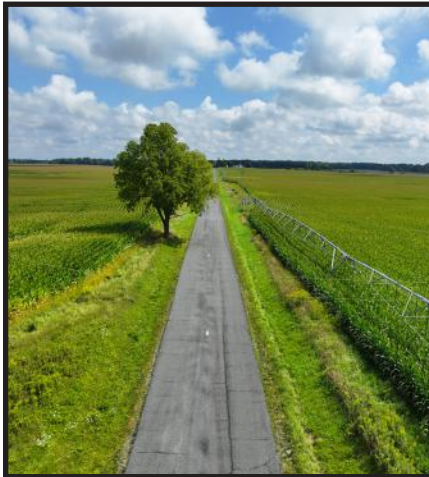
Chip seal/fog seal on OP Avenue
