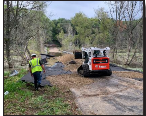
Aggregate lift on 8th Street bridge
