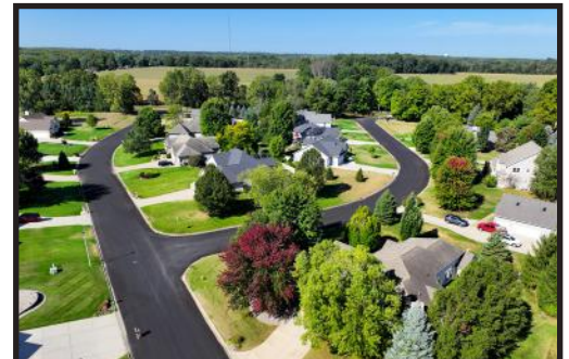
Chip seal/fog seal on Sweet Briar Drive
