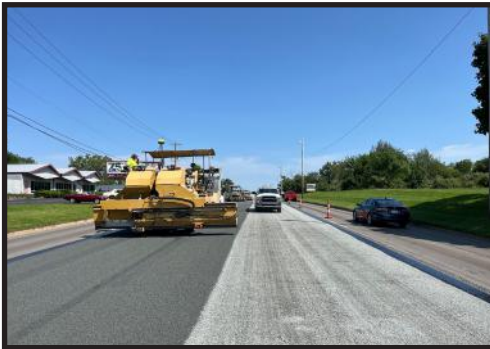
Chip seal/fog seal on Sprinkle Road
