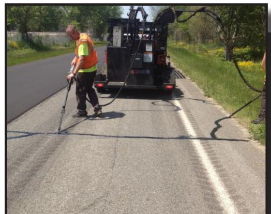
Crack fill on K Avenue
