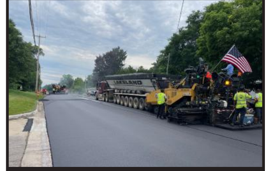
HMA paving on 9th Street
