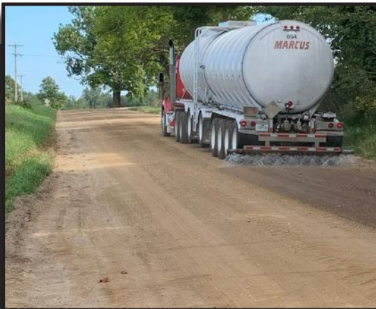
Applying dust control on 40th Street
