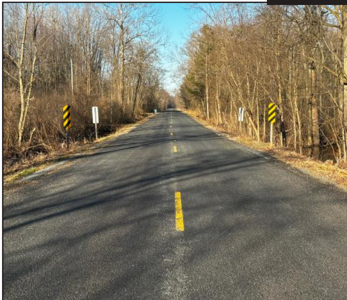
Chip seal/fog seal on AB Avenue
