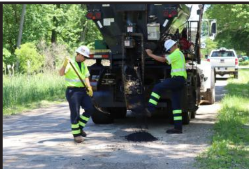
Pothole patching on AB Avenue
