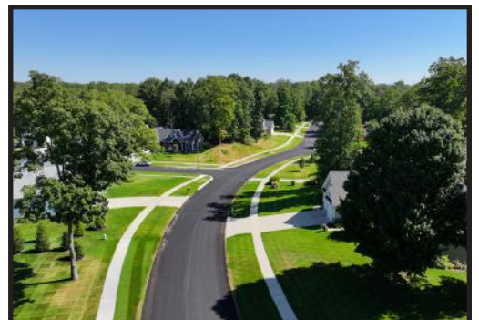
Chip seal/fog seal on Western Woods Drive
