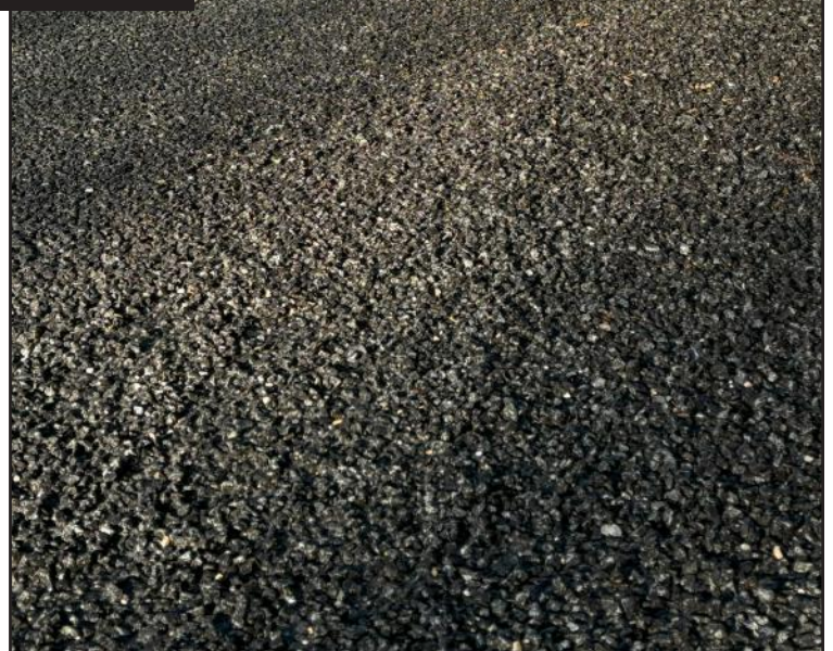
Chip seal/fog seal on AB Avenue
