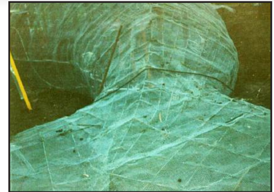
The steel armature ready to receive the first layer of render
