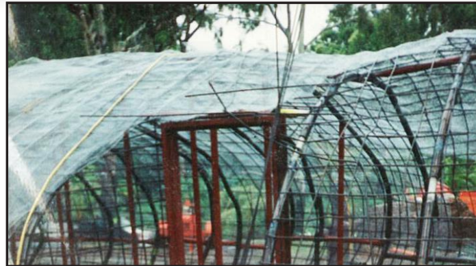
Adding the door frames & application of wire netting over 10mm mild steel bar armature. (It is built in concrete)
