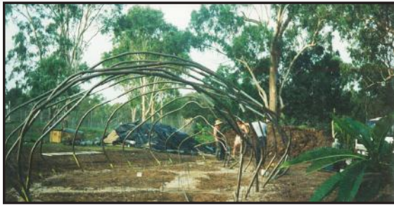
Creating the Armature - additional framing added
