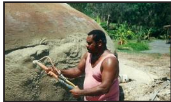
Coating with frame with Cement
