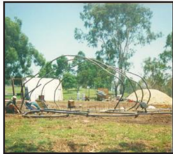
Creating the Armature - Stage 1
