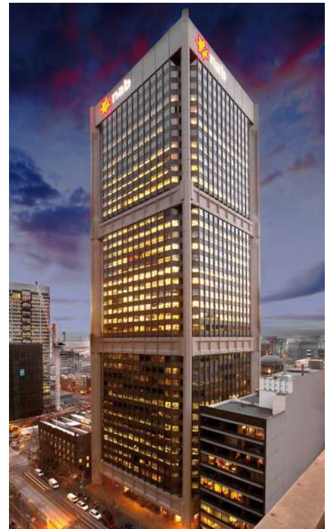
500 Bourke St, Melbourne, Australia. ISPT Operations. 5 Star Green Star - Office As Built v2. A fully electrified repositioned 1970s asset, with lower embodied carbon, and carbon neutral in operation using 100% renewable energy.
