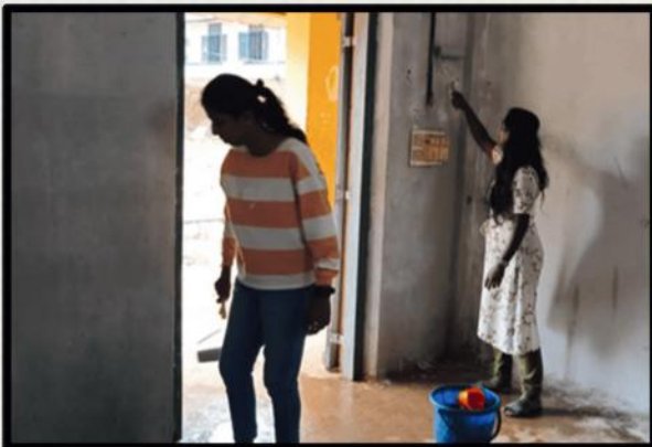
Renovation of room for NSS
