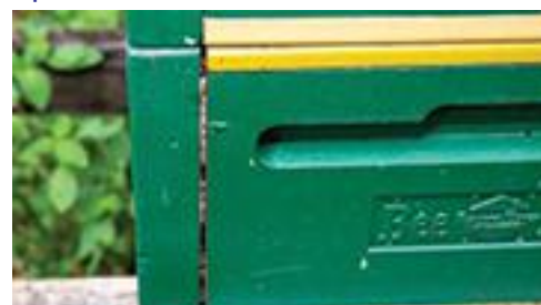
Figure 4. A cracked joint. My fault. I should have applied glue at the time of assembly.
