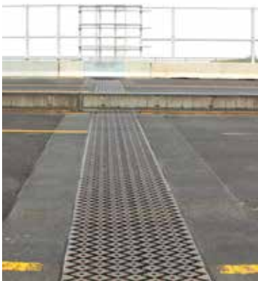
Installed expansion joint on the new bridge, which will have six lanes until the completion of the second section. Photo: MAURER
