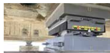
One of the 24 newly installed spherical segment bearings.
