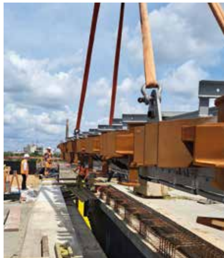
A large expansion joint is lifted into position in August 2023.
