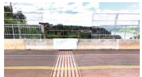
The bridge boasts the largest expansion joints ever installed in either country. These were delivered in two parts and welded together on site. Photo: Consórcio Ponte Foz
