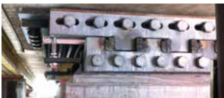
An installed bearing. During the construction phase in the launching process, temporary restraints had enabled the bearings to partially assume various functions as construction work progressed.
