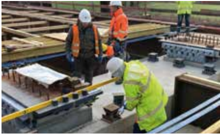
The bearings are installed on the first new bridge section in Leverkusen.
