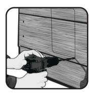
Drill 1 hole in each corner of tracing.
