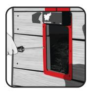
Screw in using the 6 provided screws. Leave a small space between the screw head and frame.
